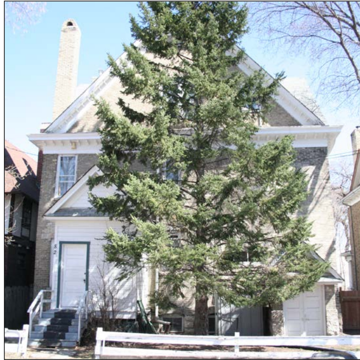
Rear (west) façade, 2007
