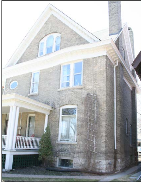
Front (east) and north façades, 2007
