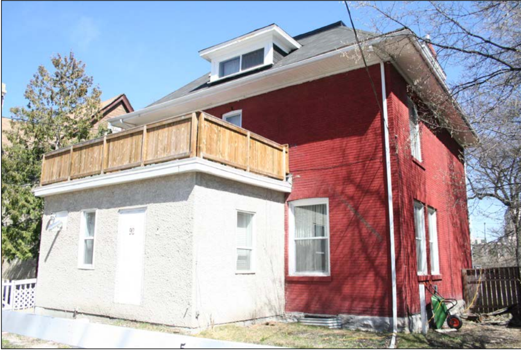
Rear (west) and south façades, 2007
