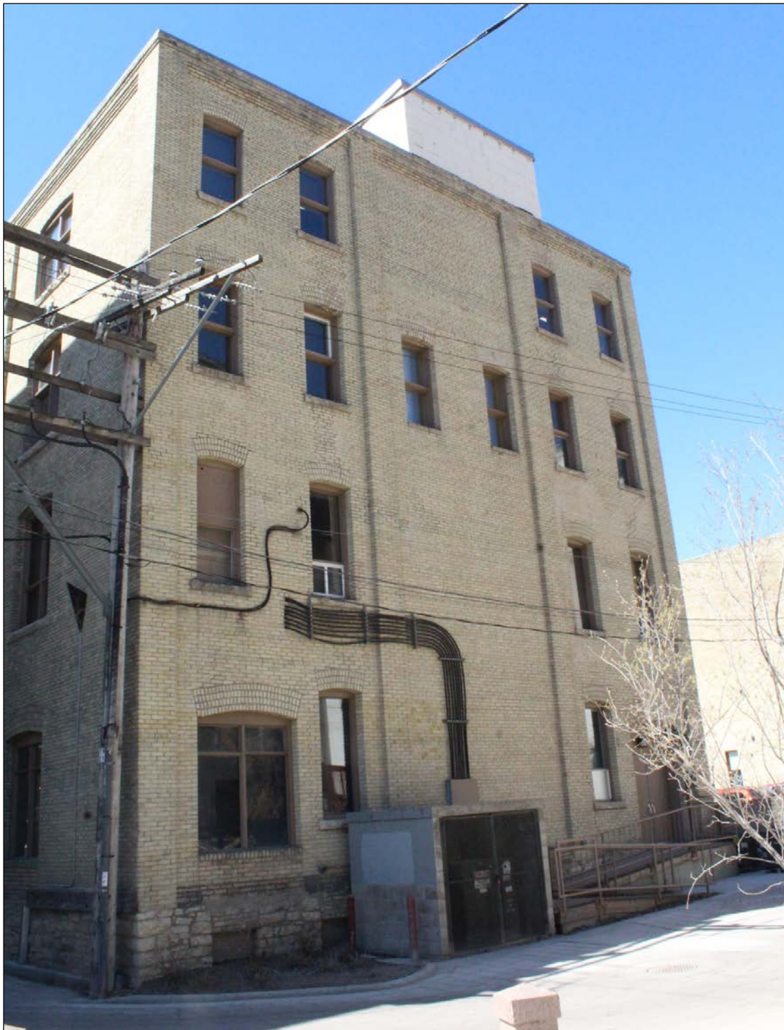
Plate 13– Marshall-Wells Warehouse, 123 Bannatyne Avenue, rear (north) façade, 2019. ( M. Peterson, 2019. )
