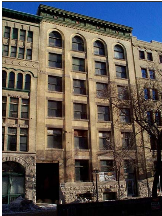
Plate 7 – Kilgour Block, 181 Bannatyne Avenue, front (south) façade. ( M. Peterson, 1999. )
