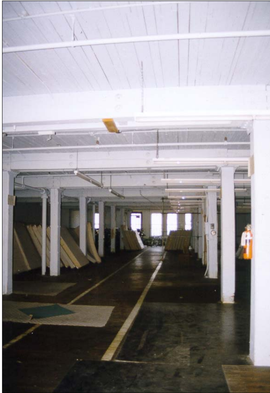
Plate 12 – Kilgour Block, 181 Bannatyne Avenue, third floor. ( M. Peterson, 1999. )
