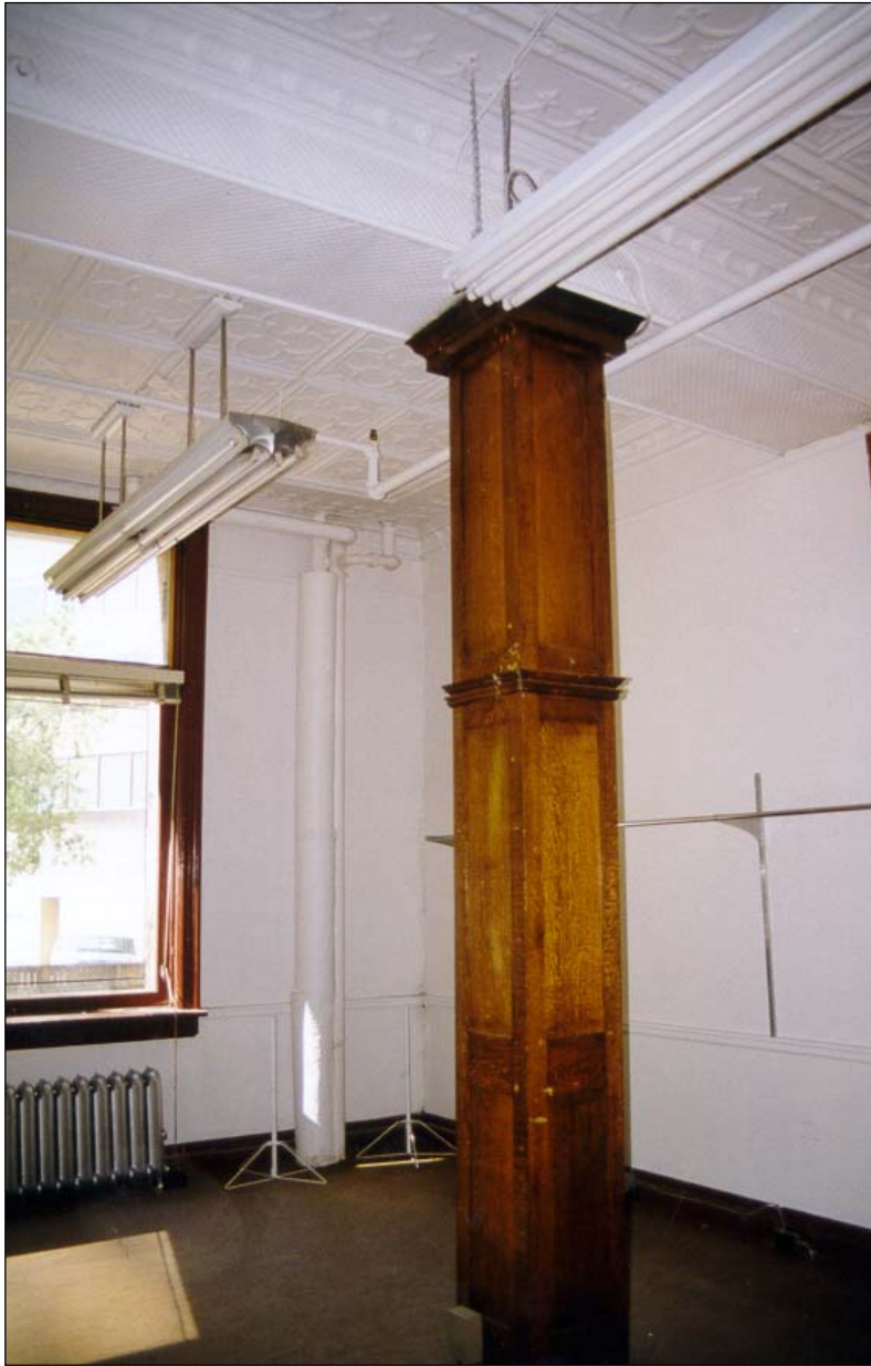
Plate 11 – Kilgour Block, 181 Bannatyne Avenue, ground floor. ( M. Peterson, 1999. )
