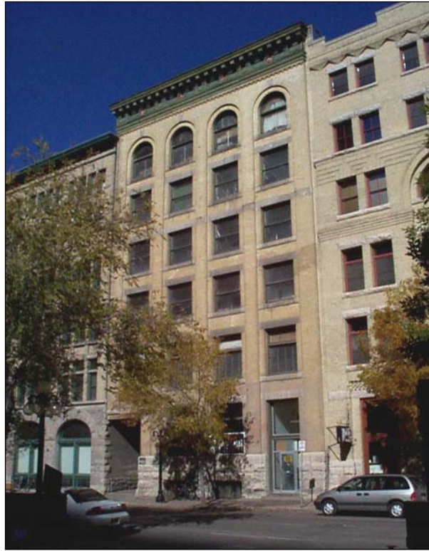
Plate 6 – Kilgour Block, 181 Bannatyne Avenue, front (south) façade. ( M. Peterson, 1998. )
