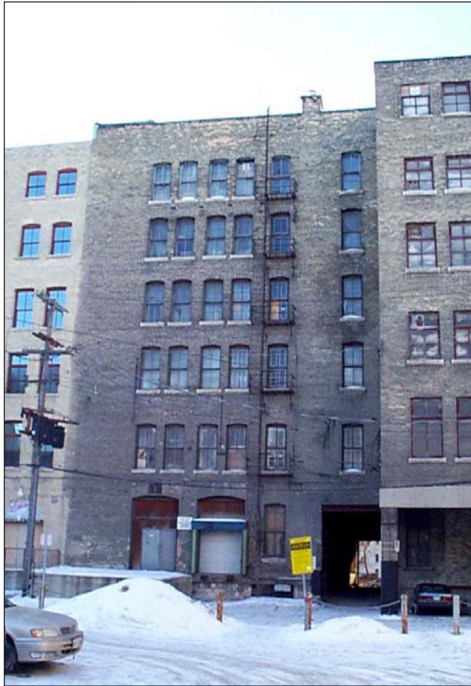
Plate 10 – Kilgour Block, 181 Bannatyne Avenue, rear (north) façade. ( M. Peterson, 1999. )
