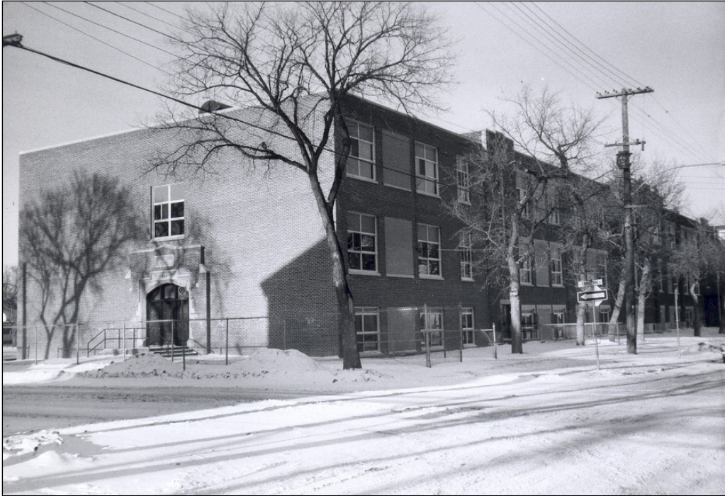
East and south façades, 1978
