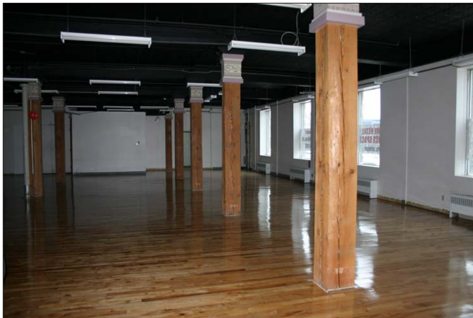
Plate 15 – Henderson Building, vacant ground-floor space. (M. Peterson, 2005.)
