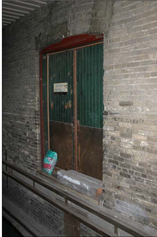
Plate 14 – Henderson Building, ground-floor loading area. (M. Peterson, 2005.)
