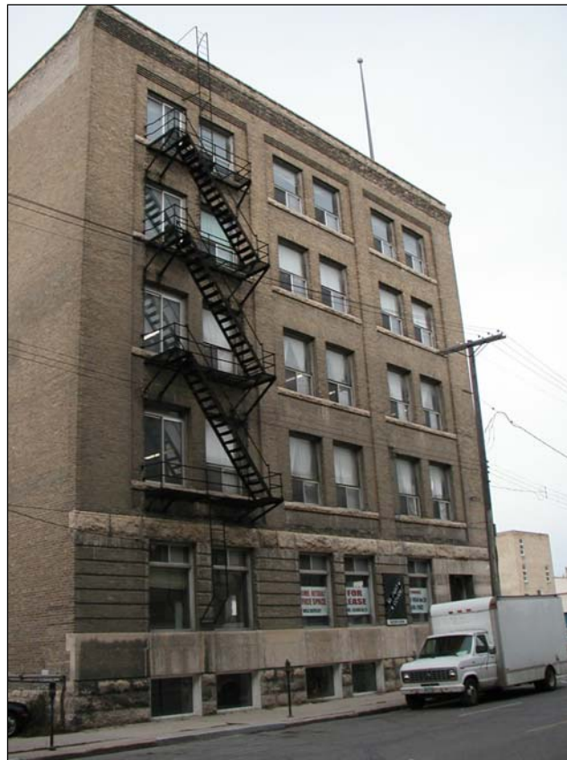
Plate 5 –Henderson Building, 332 Bannatyne Avenue, east side. (M. Peterson, 2005.)
