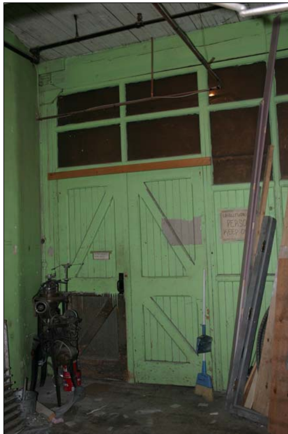
Plate 13 – Henderson Building, ground-floor loading area. (M. Peterson, 2005.)
