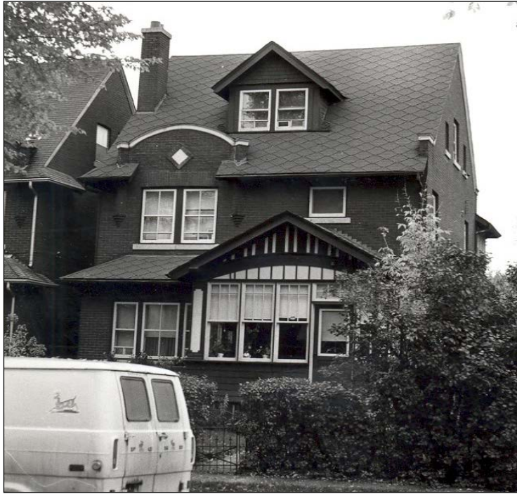
Front (south) façade, 1978
