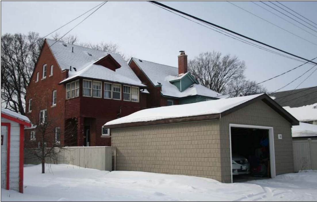
Rear (north) and east façades, 2009
