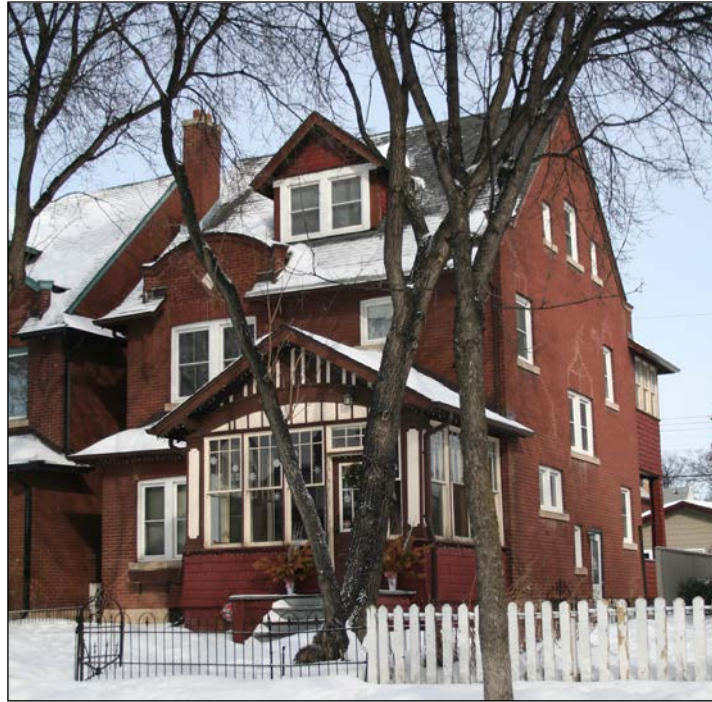
Front (south) and east façades, 2009
