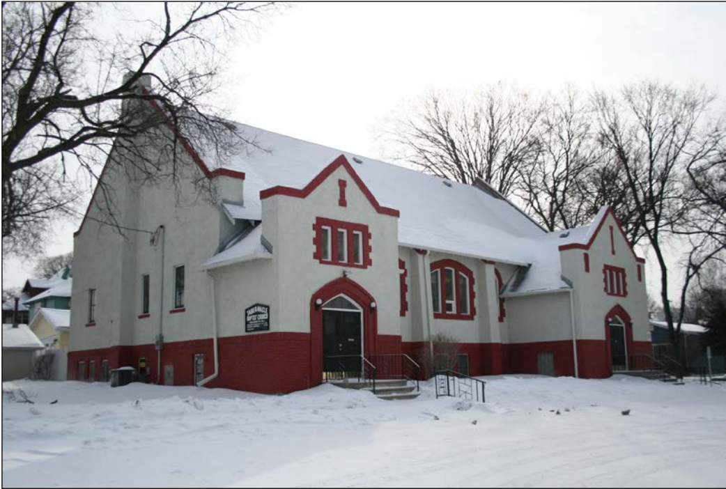
West and north façades, 2009
