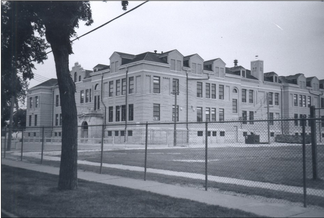
Rear (north) and east façades, 1978
