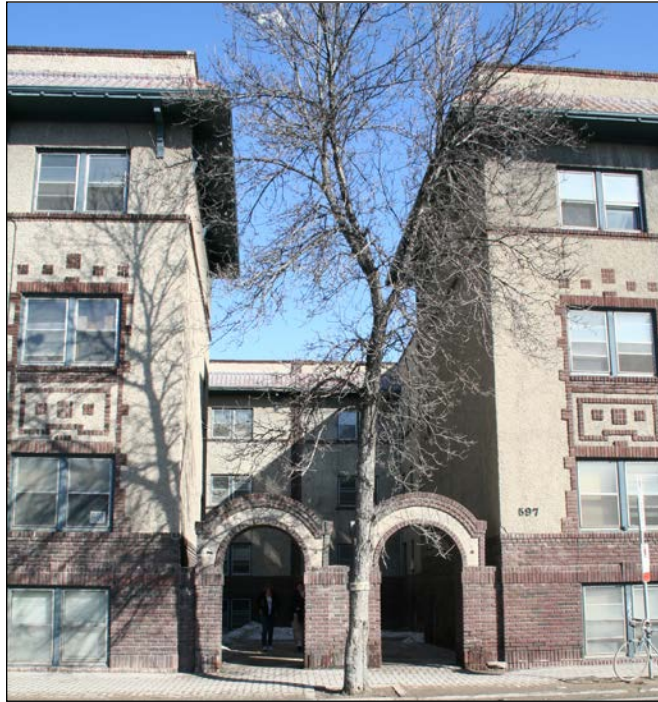
Detail of entrance to courtyard, 2009
