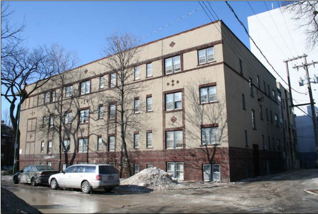
Rear (north) and east façades, 2009
