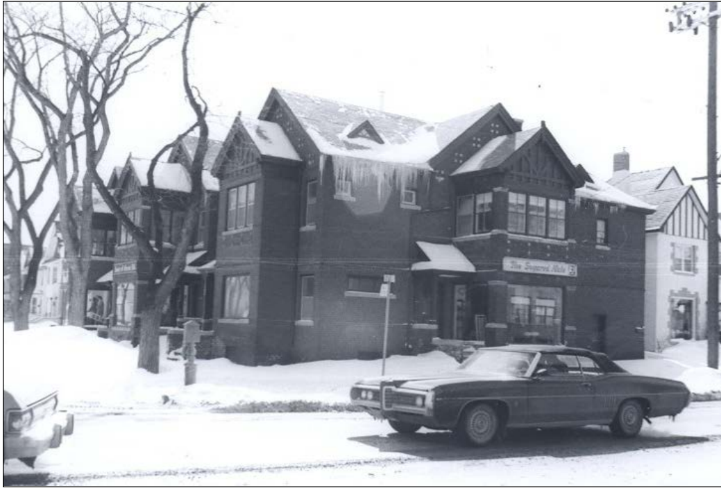
Front (north) and east façades, 1978
