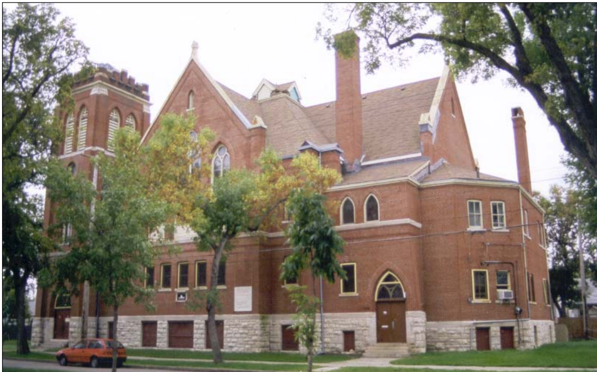
Plate 6 – Former St. Giles United Church (Presbyterian), north façade. ( M. Peterson, 1999. )
