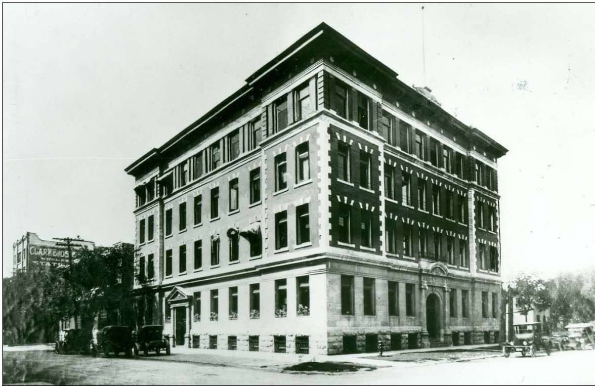
Plate 5 – Garry Telephone Exchange, 74 Charlotte Street, ca.1910. ( Archives of Manitoba, “Manitoba Telephone System Collection- 1-1”. )
