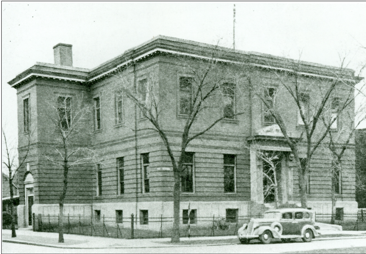
Plate 25 – St. John's Telephone Exchange, 405 Burrows Avenue, ca.1945. ( Archives of Manitoba, "Winnipeg- Buildings- Provincial- Manitoba Telephone/St. John's- 1," N9858. )
