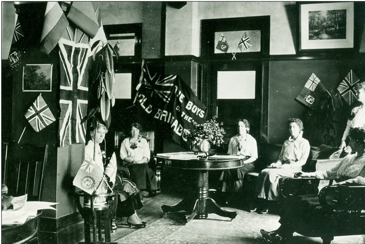
Plate 19 – Manitoba Telephone System – St. John's Exchange, 405 Burrows Avenue, first floor operators' "retiring room," ca. 1914. ( Western Canada Pictorial Index, 478-15329. )
