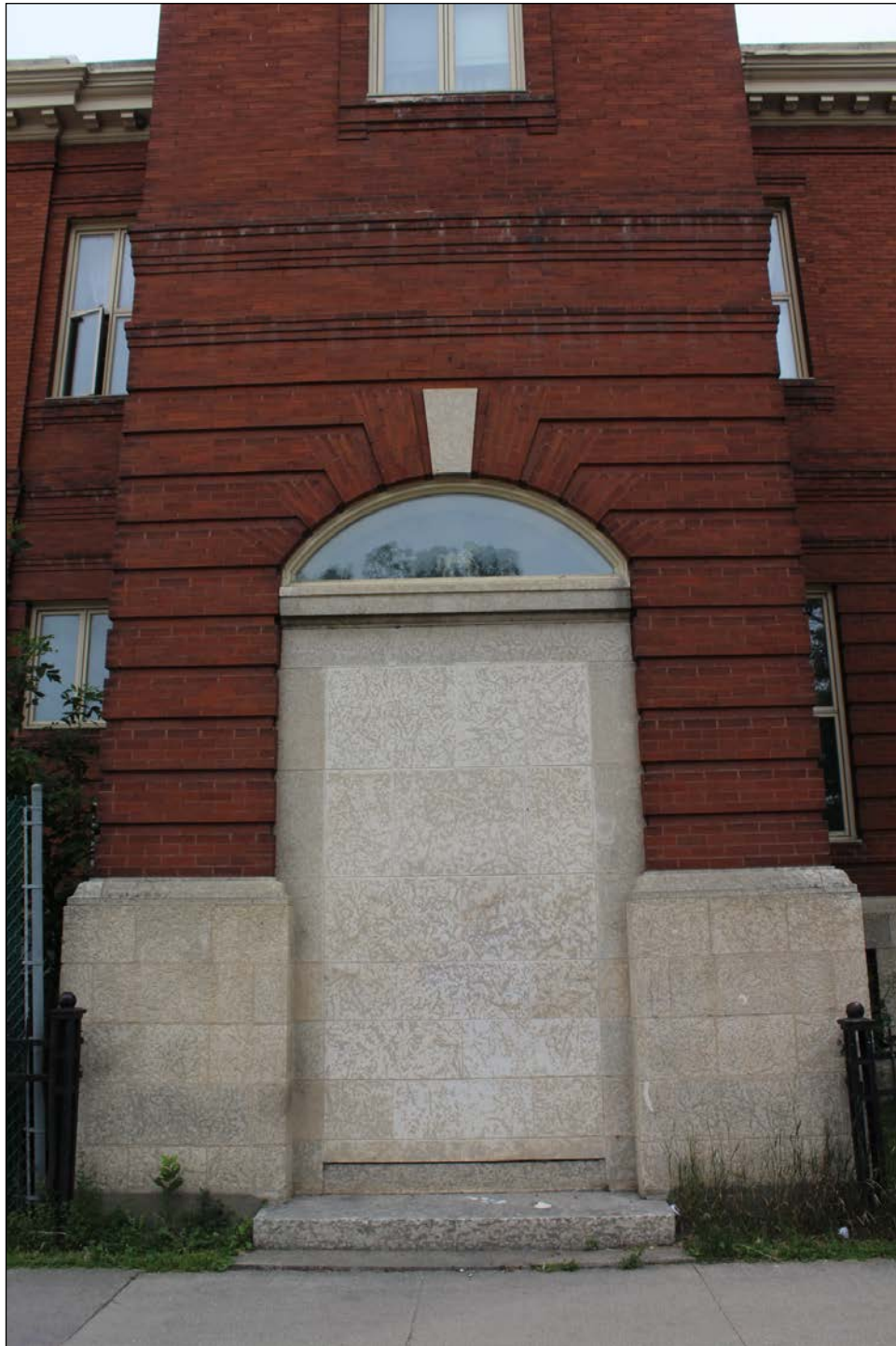
Plate 16 – Manitoba Telephone System – St. John's Exchange, 405 Burrows Avenue, west side door (now closed with stone), 2017. (M. Peterson, 2017.)
