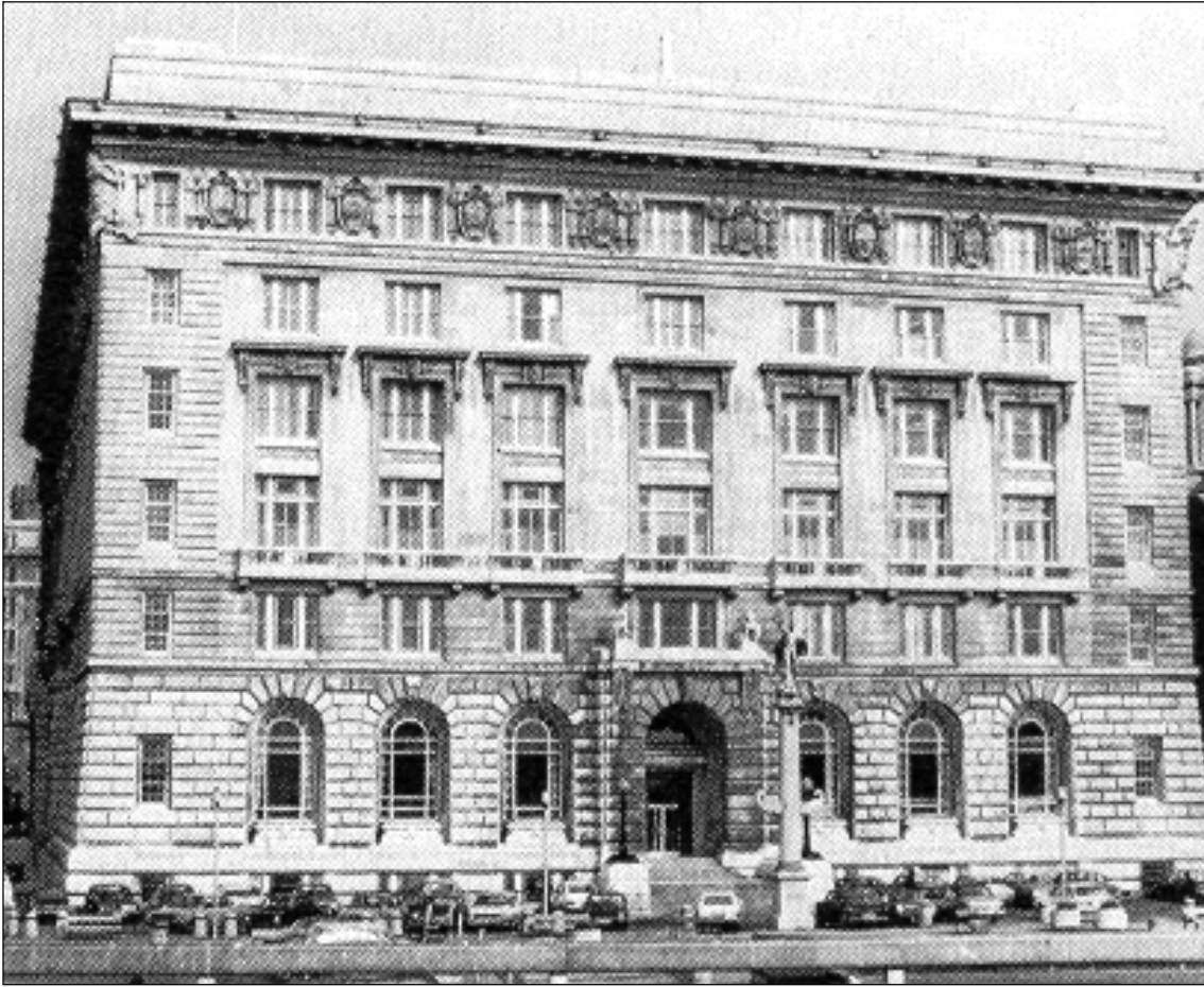
Plate 5 – Cunard Building, Liverpool, England, 1914-16; designed by Mewès and Davis. A good example of the muted ornamentation of the post-1906 Baroque Revival school. (Reproduced from A. Service, Edwardian Architecture (London: Thames and Hudson, 1977), p. 185.)
