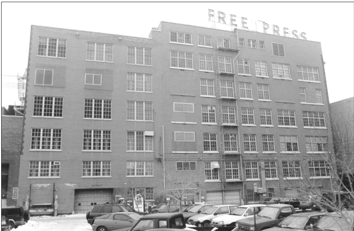
Plate 9 – Free Press Building, 300 Carlton Street, rear (west) façades of 1911-13 and 1926 buildings. ( Murray Peterson, 1998. )
