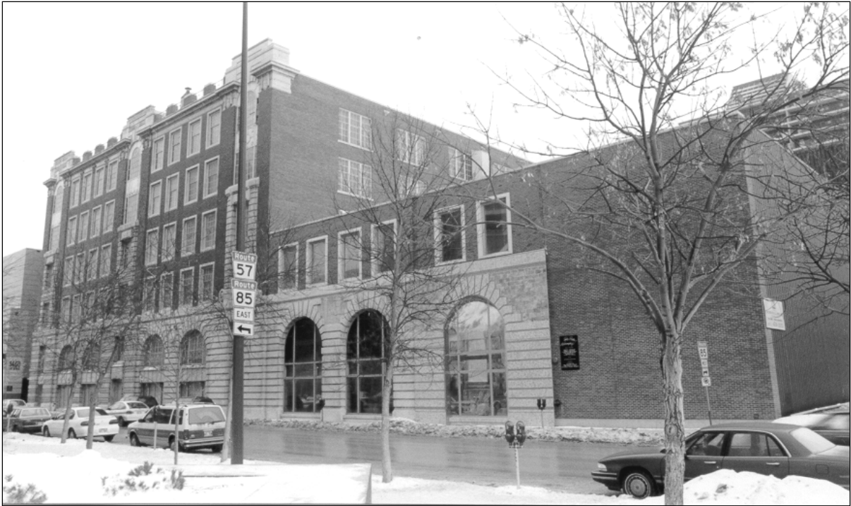
Plate 8 – Free Press Building, 300 Carlton Street, front (east) façade. ( Murray Peterson, 1998. )
