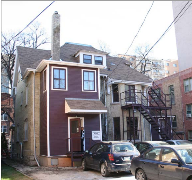
Rear (west) and north façades, 2006
