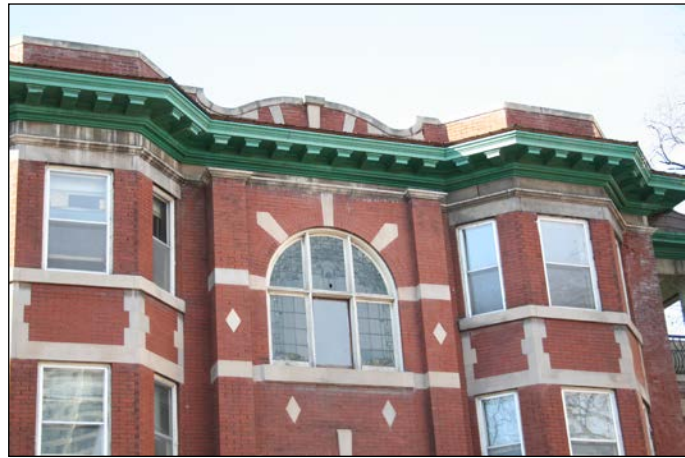
Front (east) façade details, 2006
