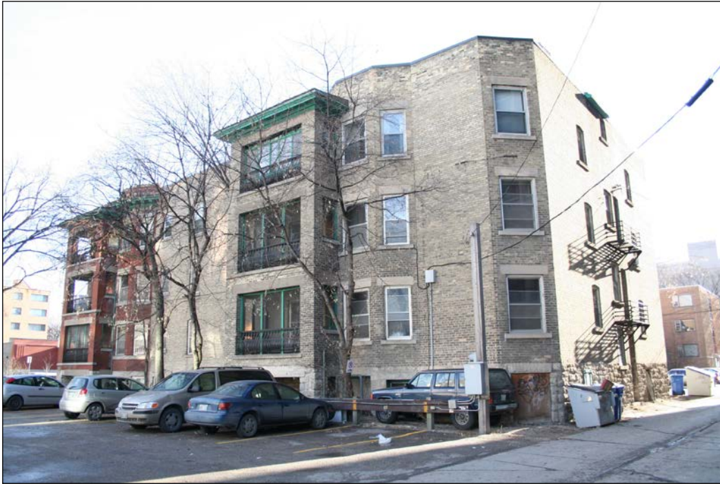
Rear (west) and north façades, 2006
