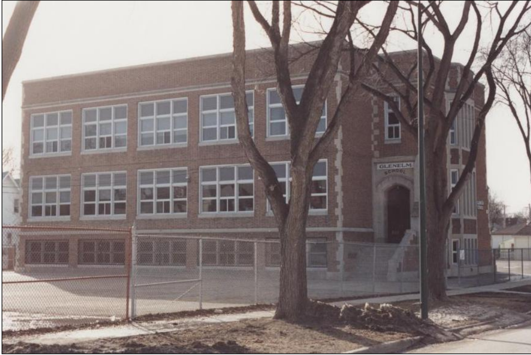
Front (north) and east façades, 1997
