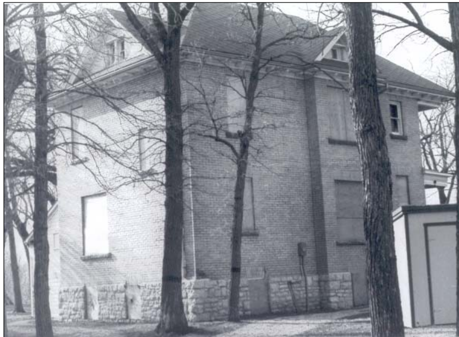
Plate 4 – Rear (south) and east façades, no date. (Courtesy of the City of Winnipeg, Planning Department. )
