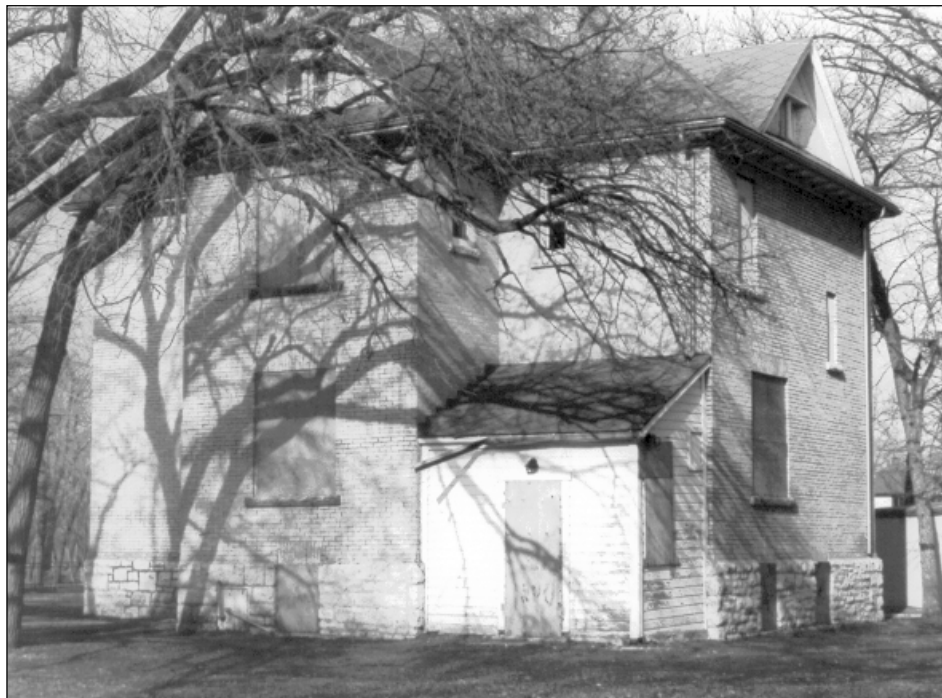
Plate 6 – Rear (south) and west façades, no date. (Courtesy of the City of Winnipeg, Planning Department.)
