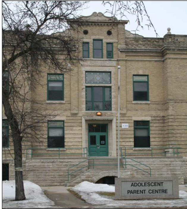
Front (east) façade detail, 2009
