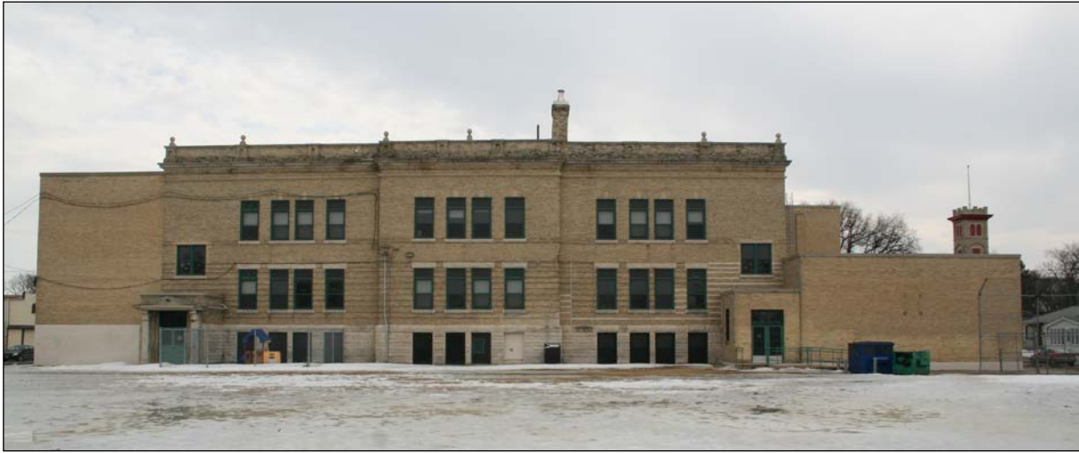
Rear (west) façade, 2009
