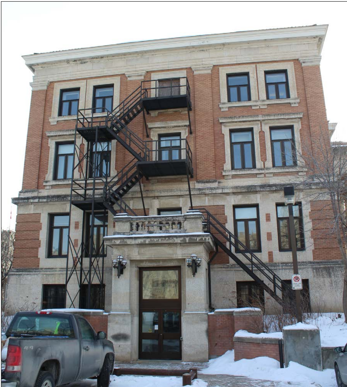
Plate 16 – University of Manitoba (Manitoba Agricultural College) Administration Building, 66 Chancellors Circle, north façade, 2018. (M. Peterson, 2018.)
