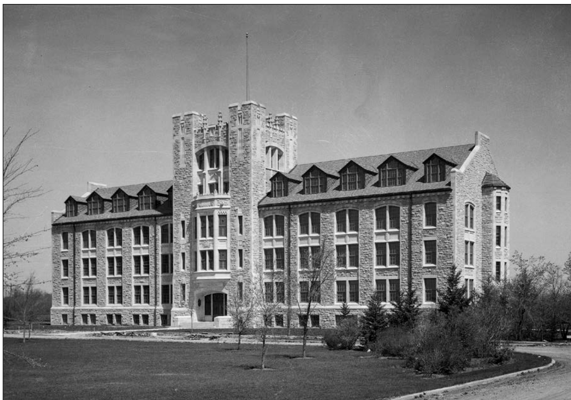
Plate 26 – Tier Building, University of Manitoba Fort Garry Campus, 1935. ( M. Peterson Collection. )
