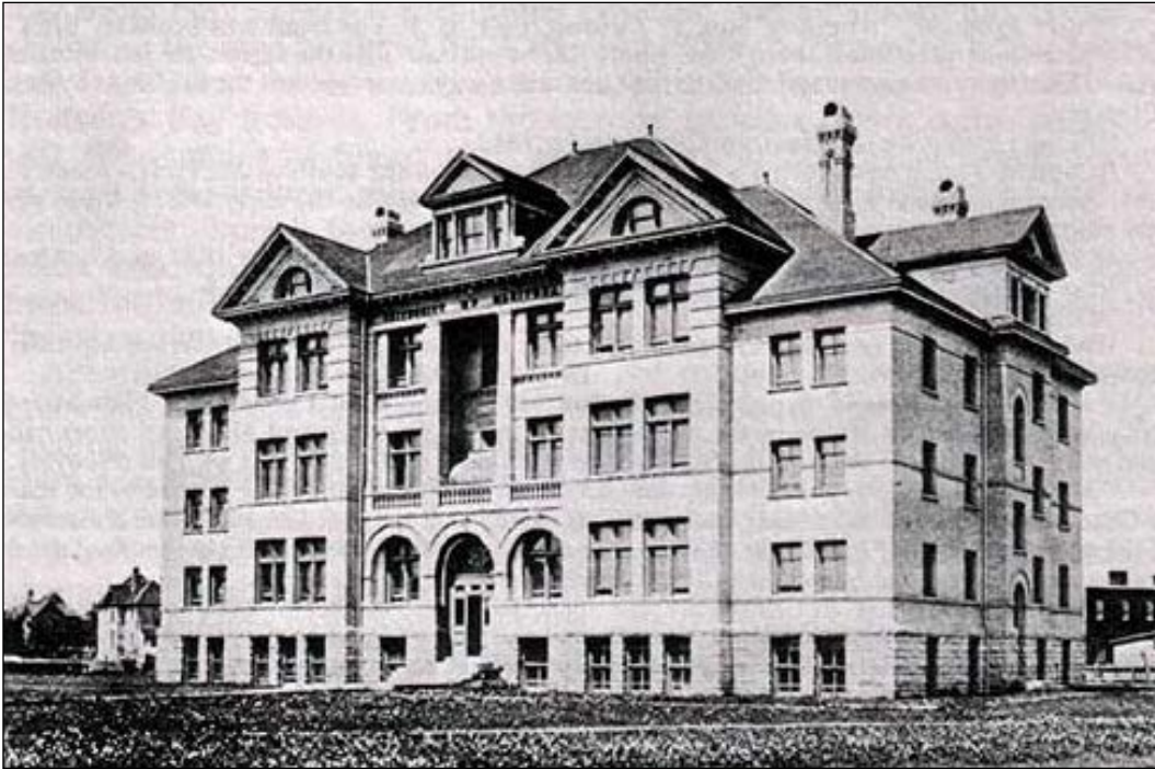
Plate 24 – University of Manitoba, Science Building (built 1900-1901), Broadway near the present-day Law Courts Building and Provincial Land Title Building, 1910. (Reproduced from Manitoba Pageant, Autumn 1977, Vol. 23, No. 1.)
