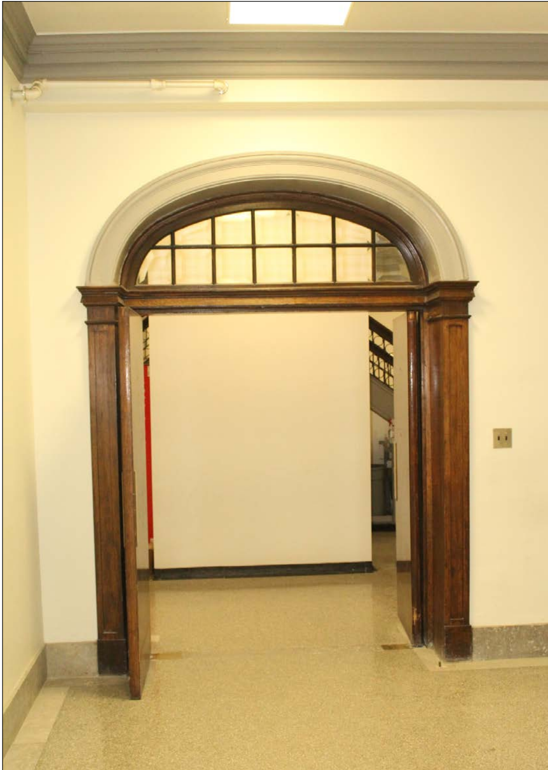
Plate 17 – University of Manitoba (Manitoba Agricultural College) Administration Building, 66 Chancellors Circle, doorway with wood trim and multi-paned arched transom, 2017. ( M. Peterson, 2017. )
