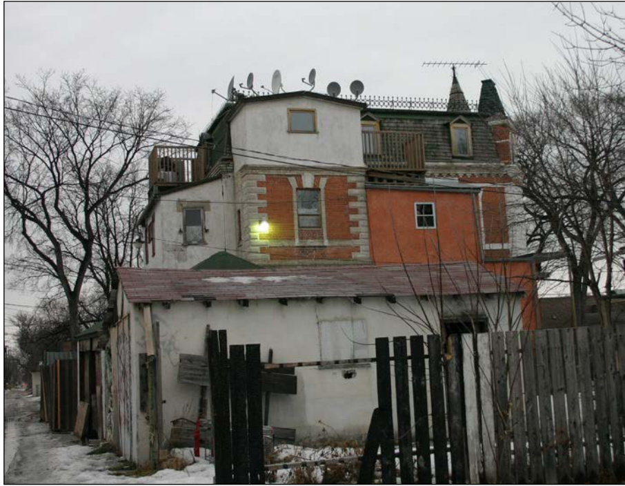
Rear (south) and east façades, 2009
