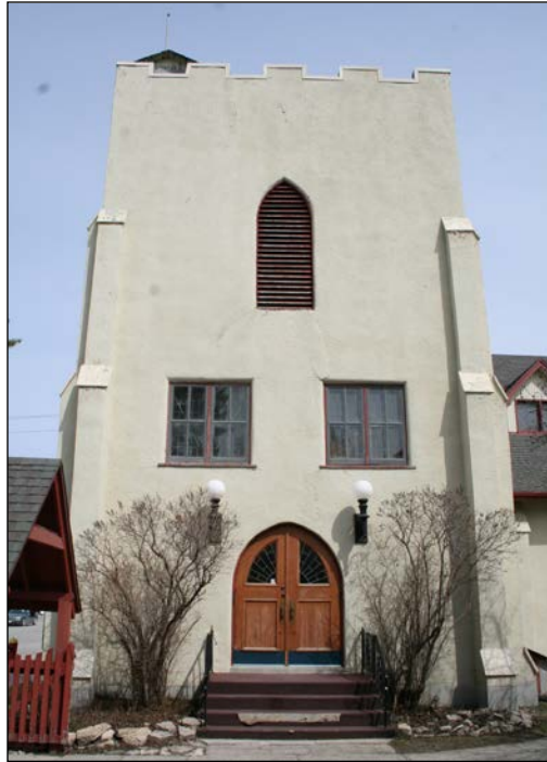
East façade detail, 2009
