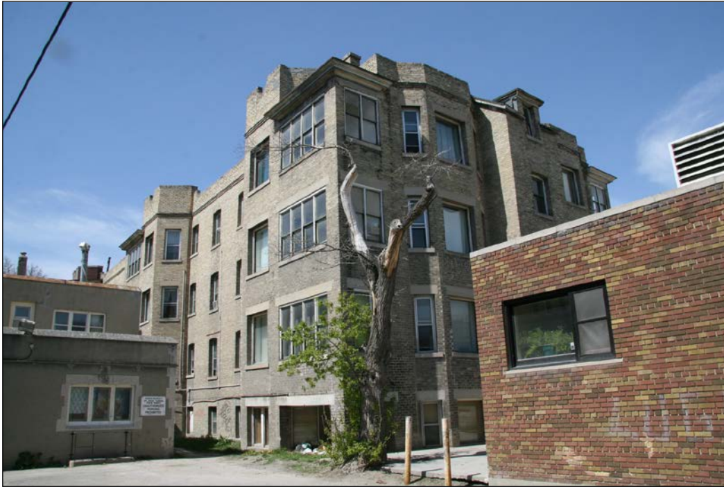
Rear (east) and south façades, 2007
