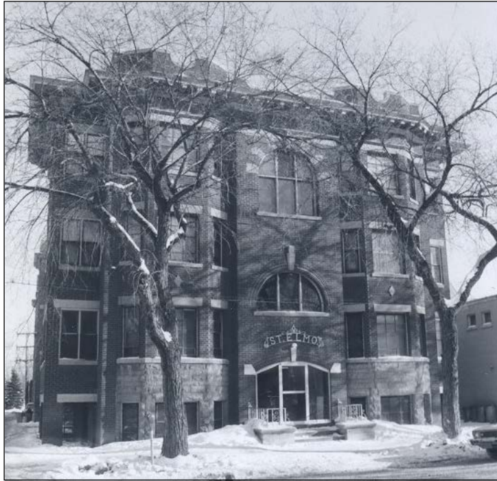
Front (west) façade, 1978
