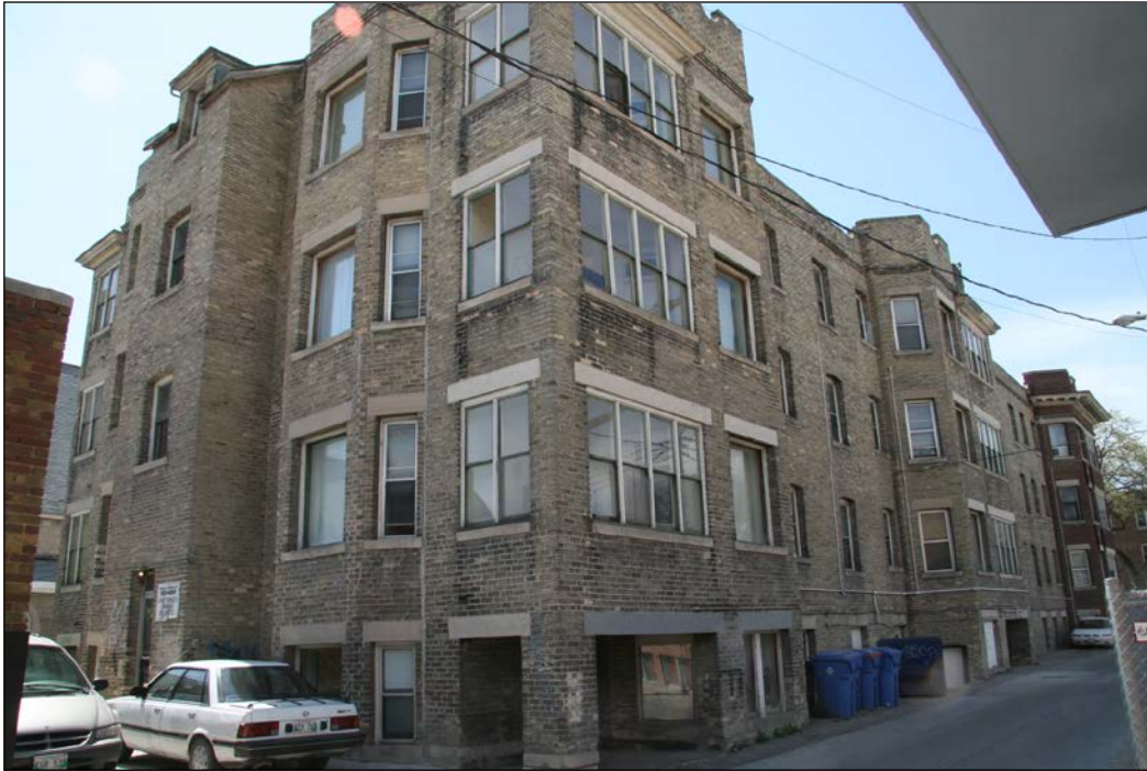
Rear (east) and north façades, 2007
