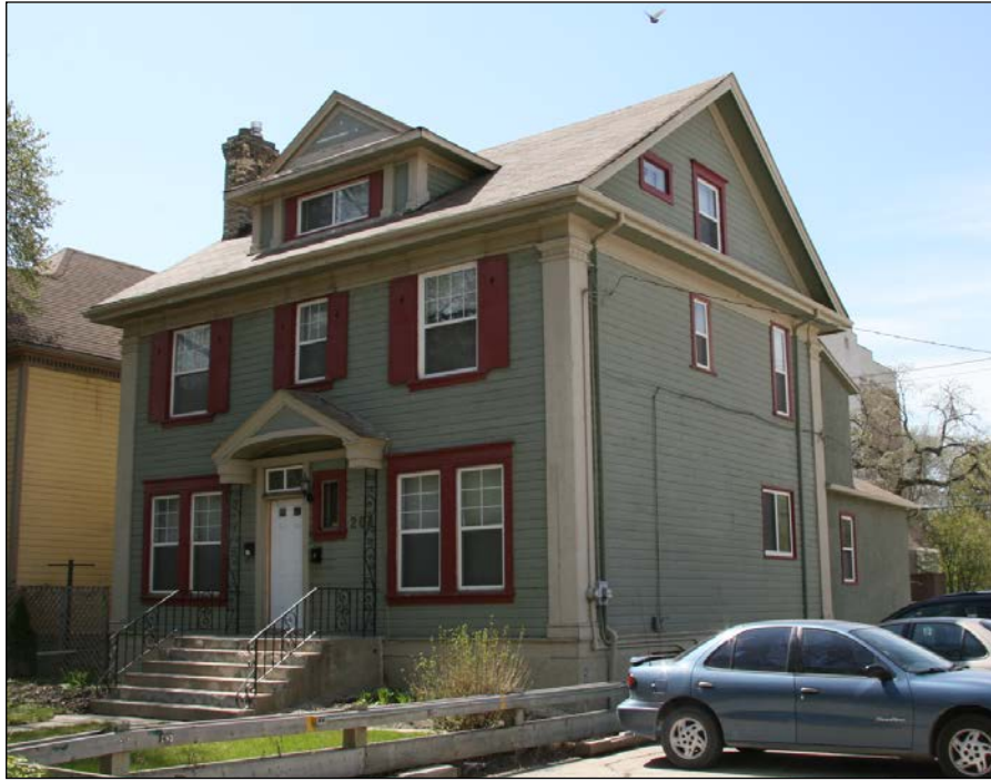
Front (east) and north façades, 2007
