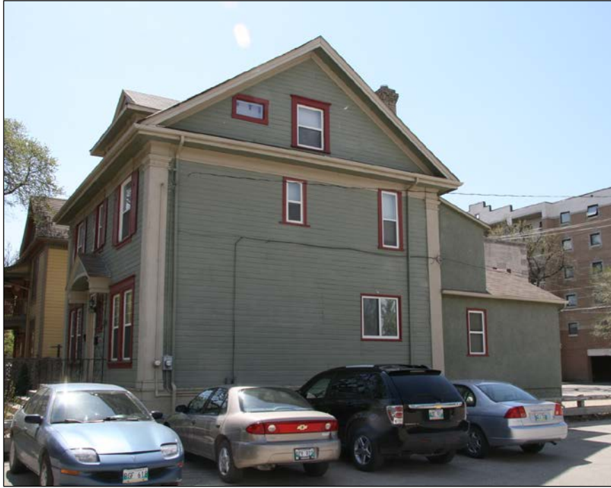
Front (east) and north façades, 2007
