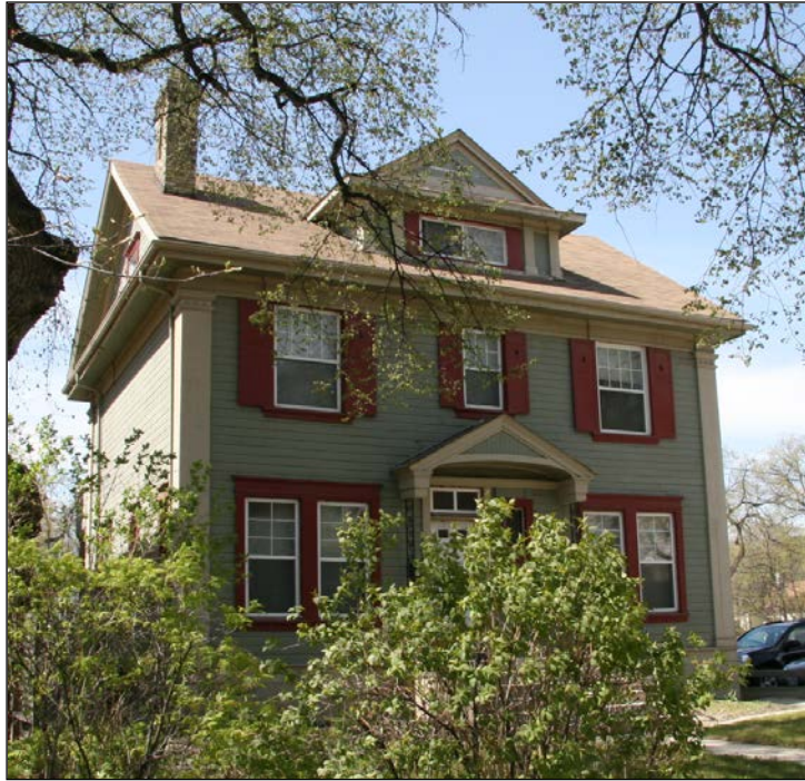
Front (east) and south façades, 2007
