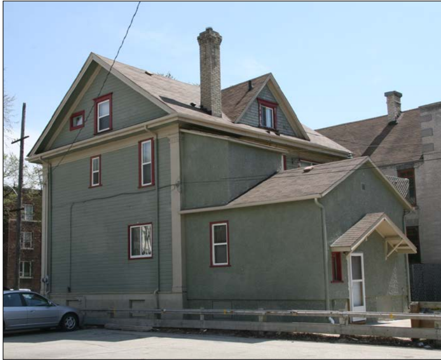
Rear (west) and north façades, 2007
