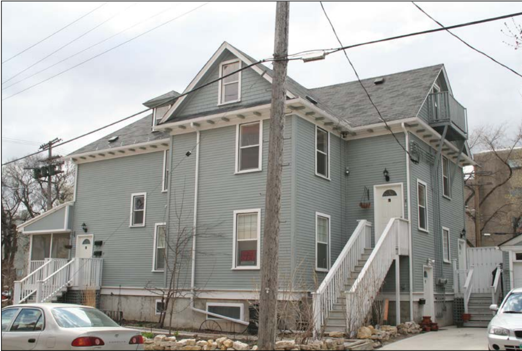
Rear (north) and east façades, 2009
