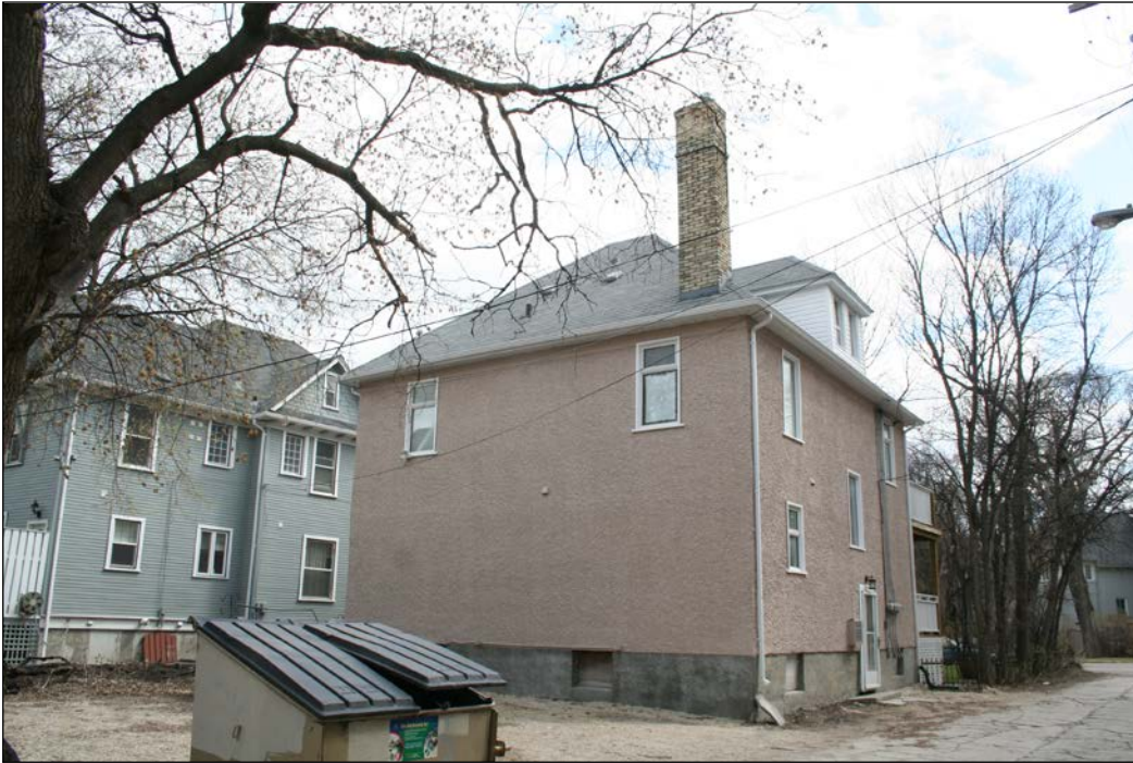
Rear (north) and west façades, 2009
