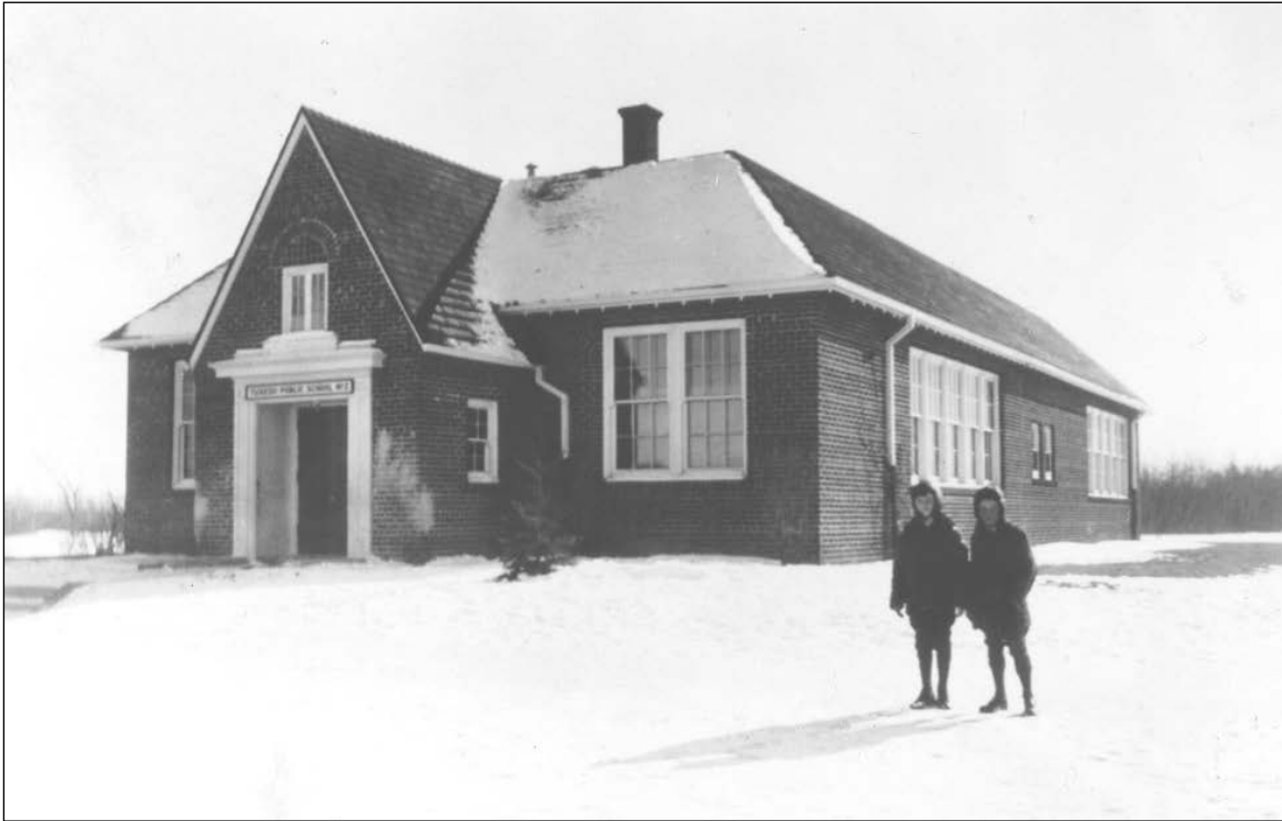
Plate 4 – Tuxedo Public School No. 2, 1939. Notice the large, multi-paned windows on the front and side elevations. ( Provincial Archives of Manitoba, Peter McAdam Collection, #341. )
