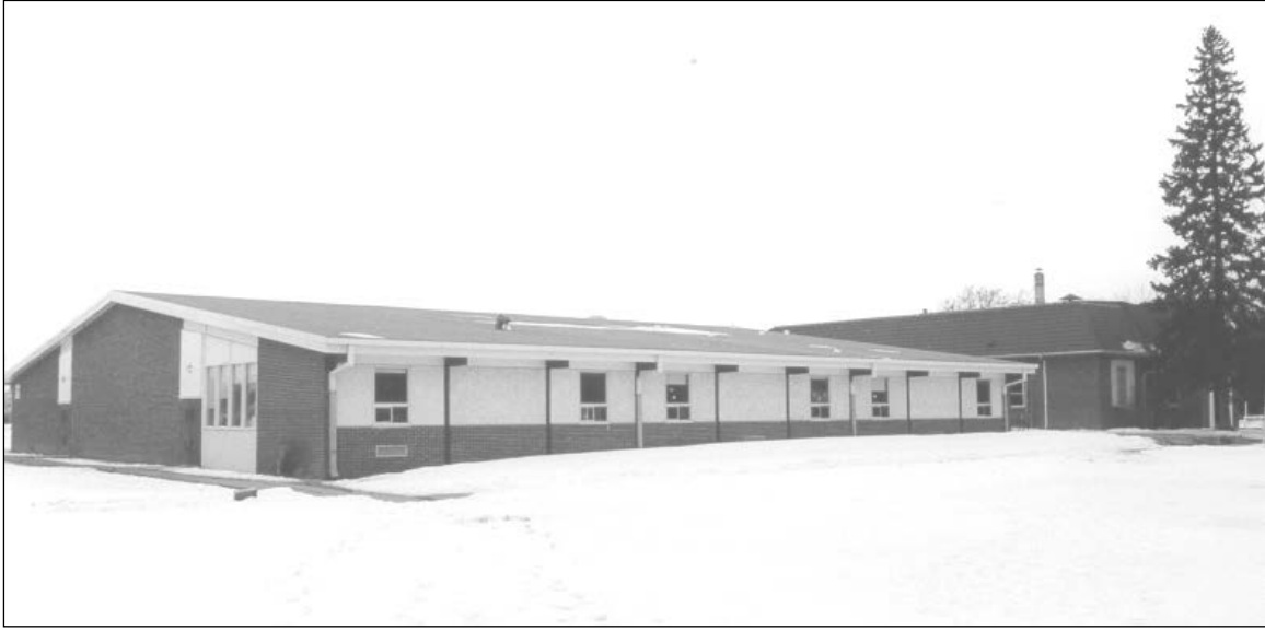
Plate 6 – Tuxedo School, 1957 and 1959 additions. ( M. Peterson, 1998. )
