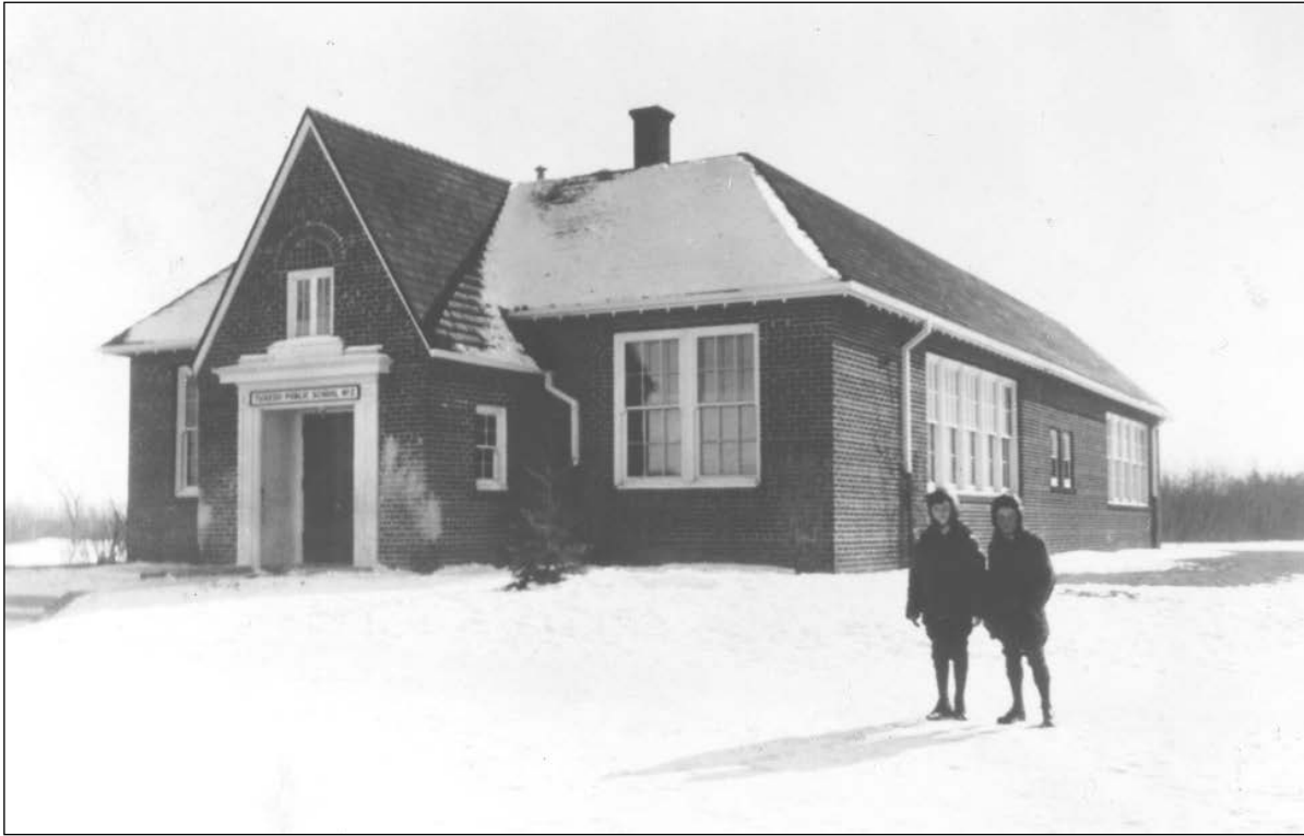
Plate 3 – Tuxedo Public School No. 2, 1939. Notice the large, multi-paned windows on the front and side elevations. ( Provincial Archives of Manitoba, Peter McAdam Collection, #341. )
