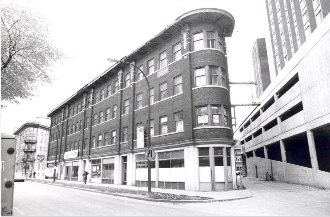
Nakomis Building, 1978. Note the original brick doorframes on the ground floor.
