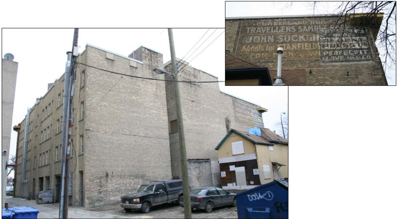
Rear (south) and east façades and east side painted signage, 2006.
