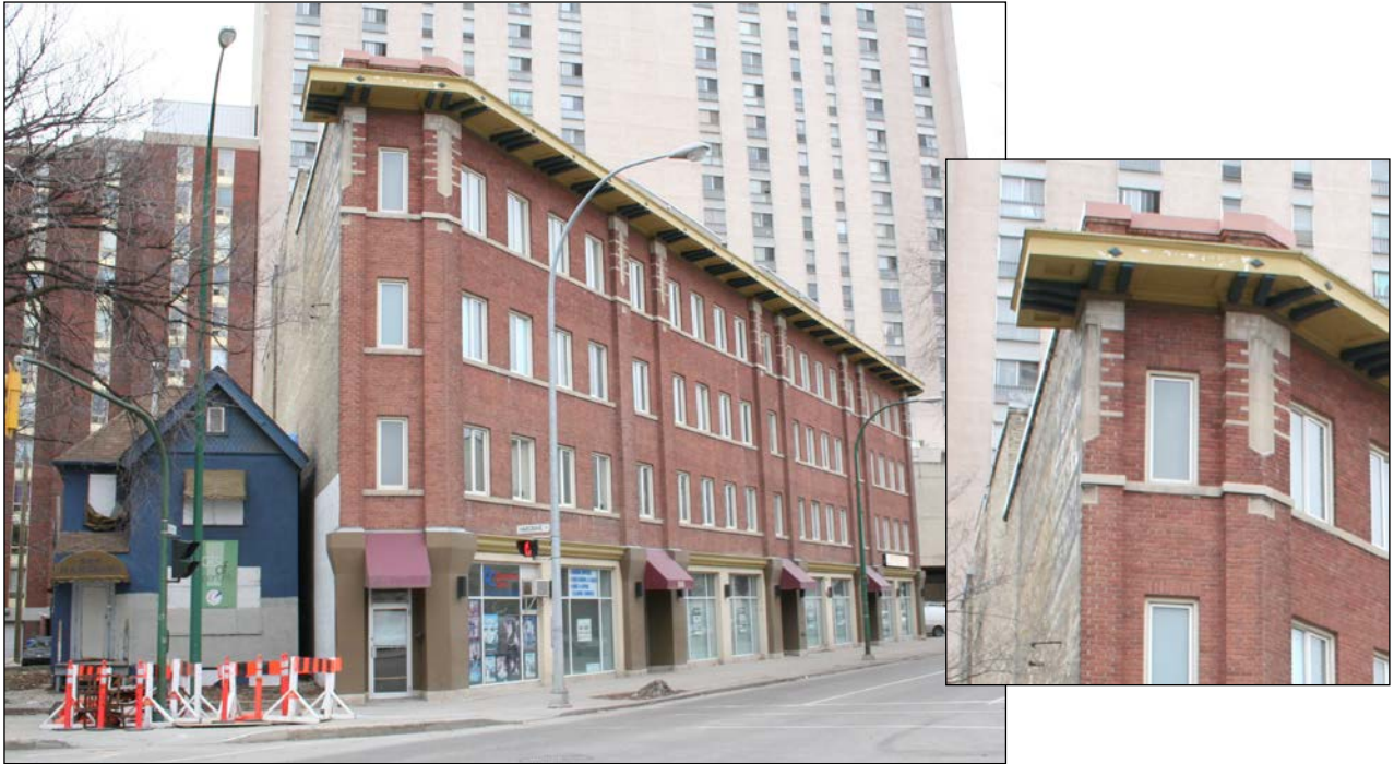
Front (north) and east façades and northeast corner detail, 2006.
