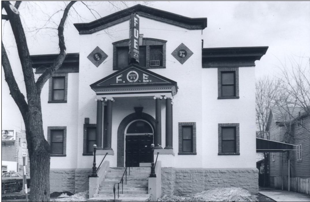
Front (west) façade without north and south additions, 1978
