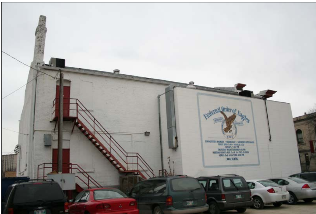
North side façade, 2006
