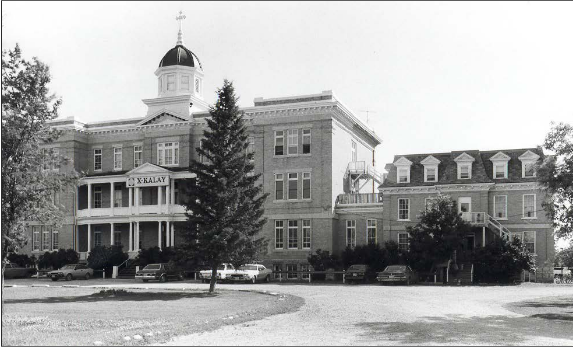
Front (west) façade, 1983
