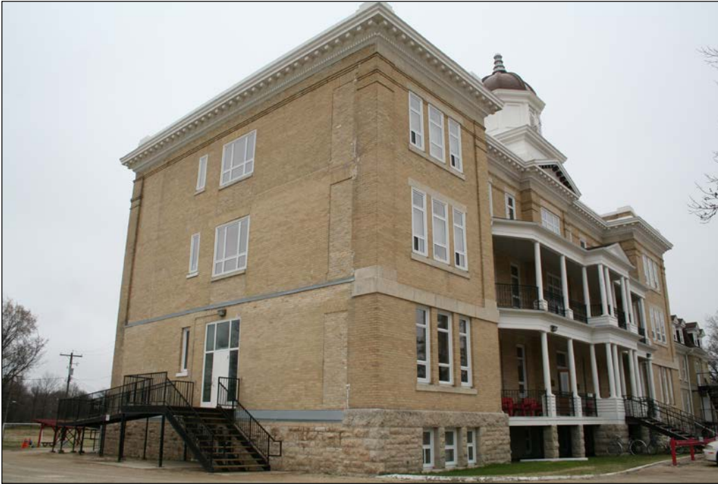
Front (west) and north façades, 2009
