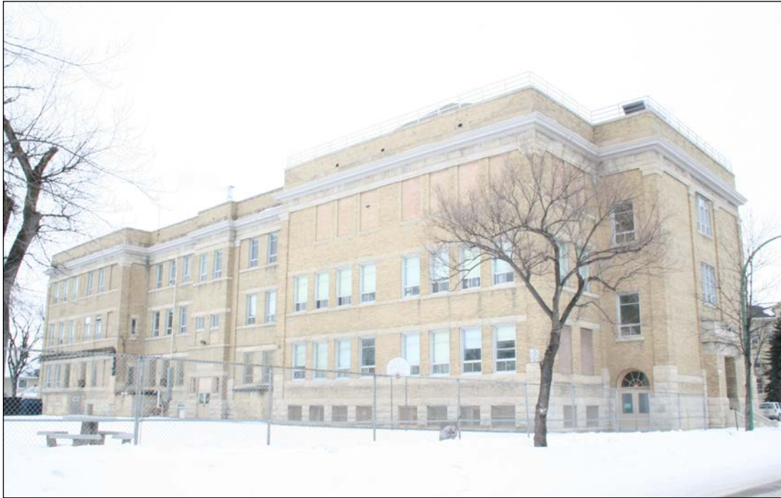
Rear (south) and east façades, 2009
