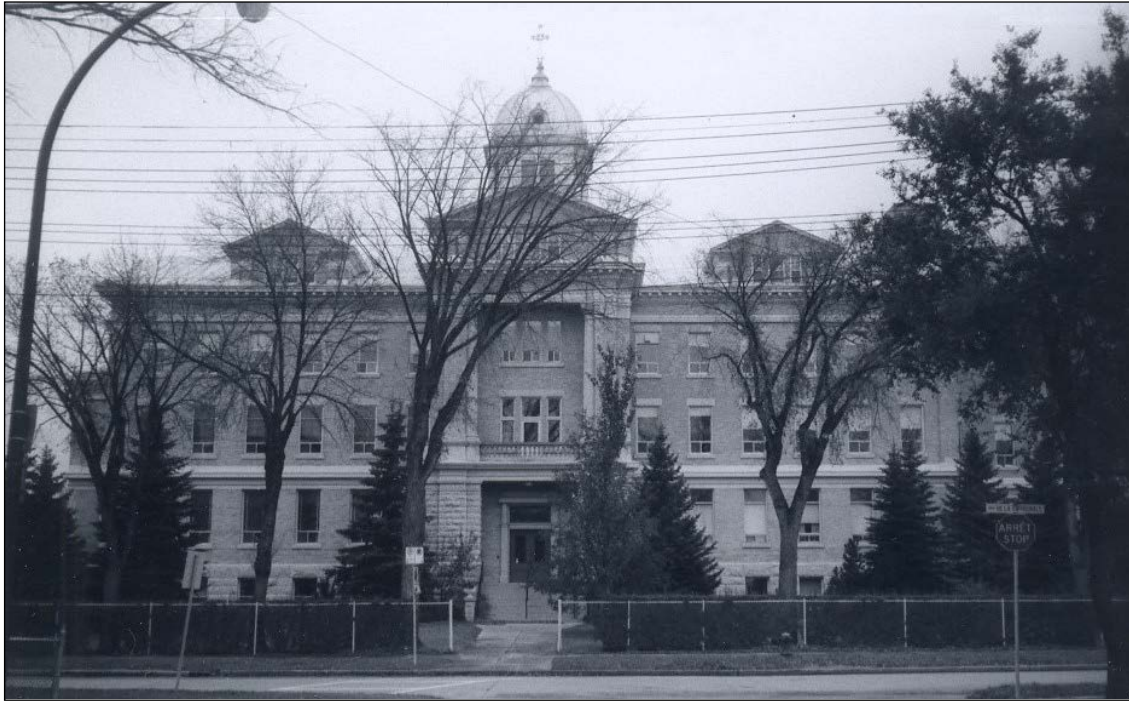
Front (south) façade, 1978
