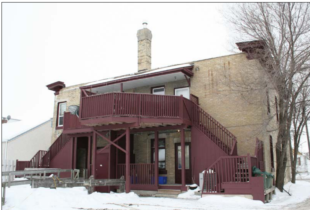
Rear (east) and north façades, 2009
