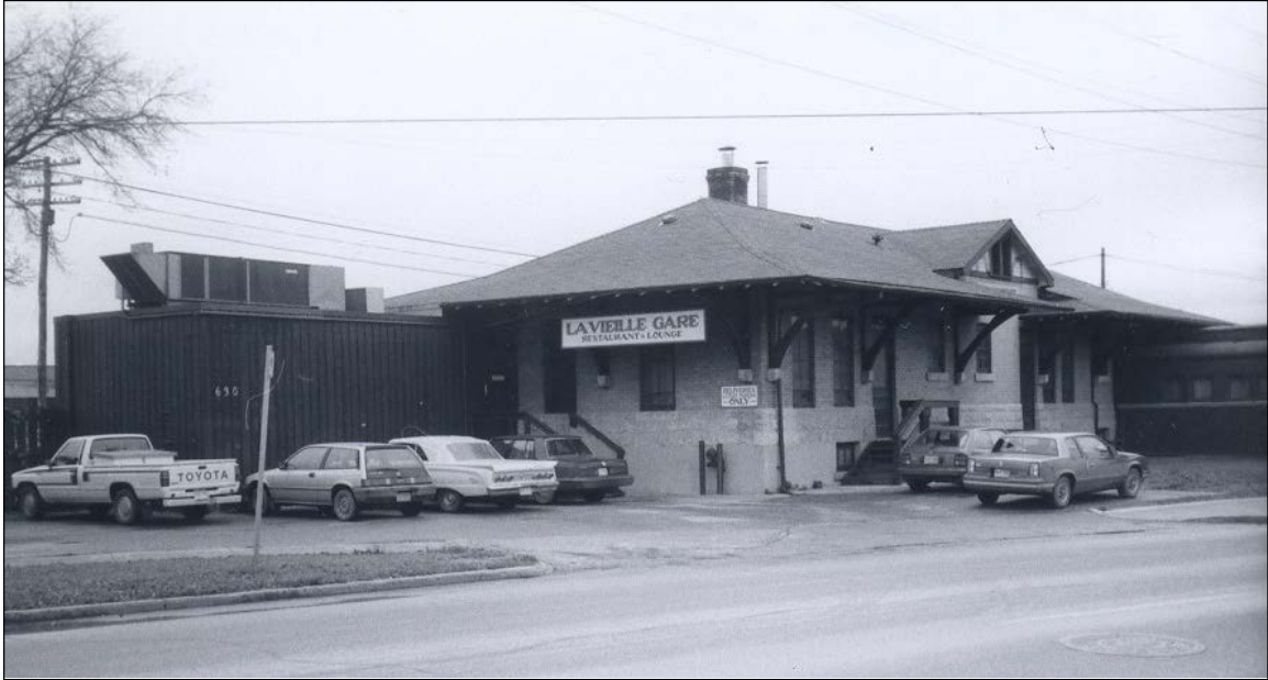
Front (west) façade, 1978
