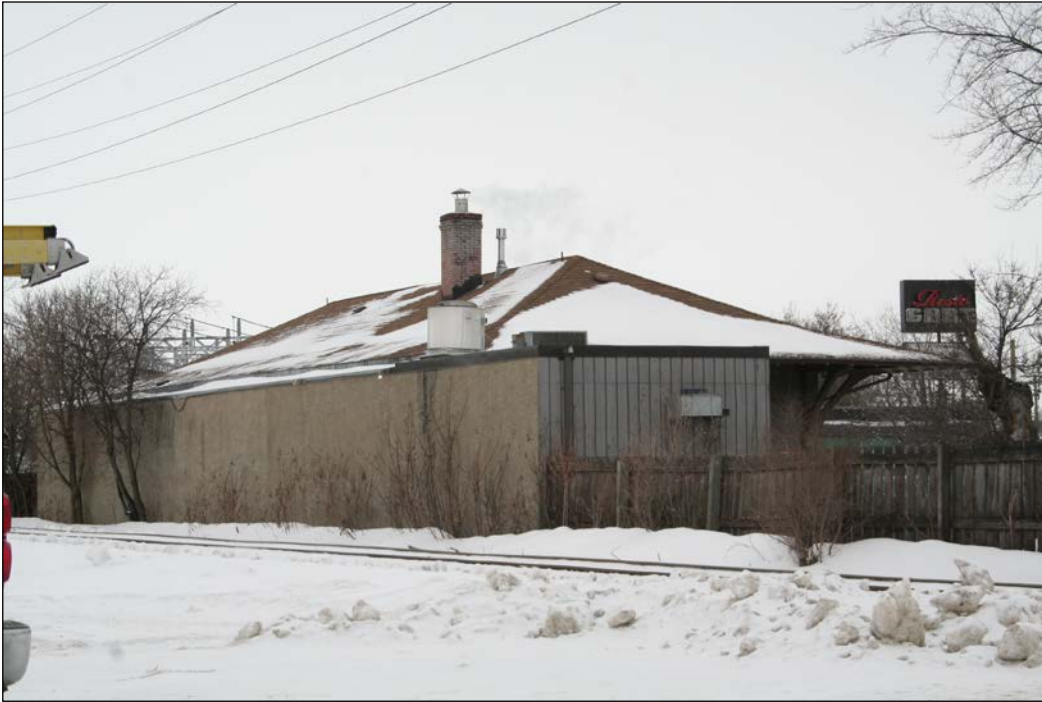
Trackside (east) and north façades, 2009
