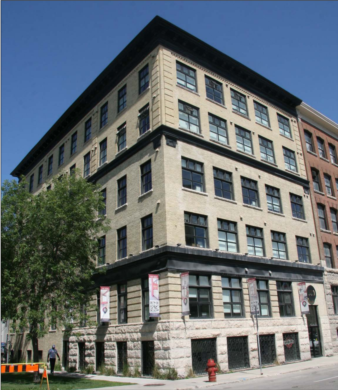
Plate 13 – Bell Block, 370 Donald Street, front (east) and south façades, 2015. ( M. Peterson, 2015. )
