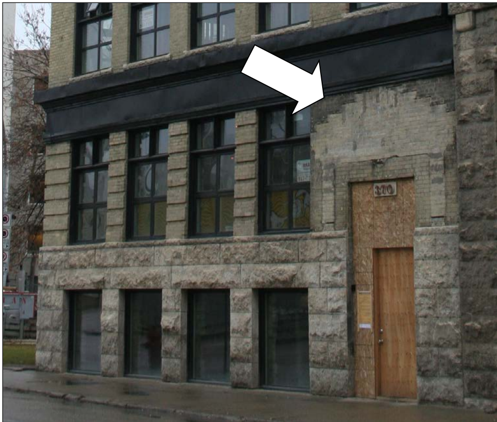
Plate 12 – Bell Block, 370 Donald Street, detail of ground floor, including outline of original pediment (arrow), 2012. (M. Peterson, 2012.)
