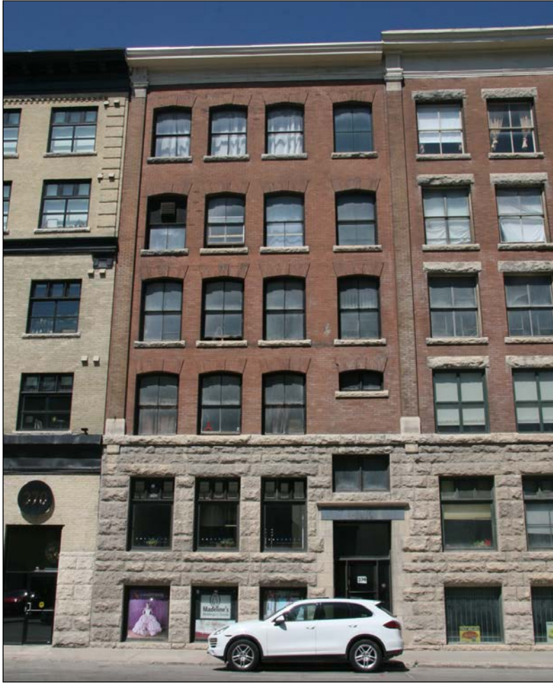
Plate 9 – Aldous Building, 376 Donald Street, south end of the front (east) façade, 2015. ( M. Peterson, 2015. )
