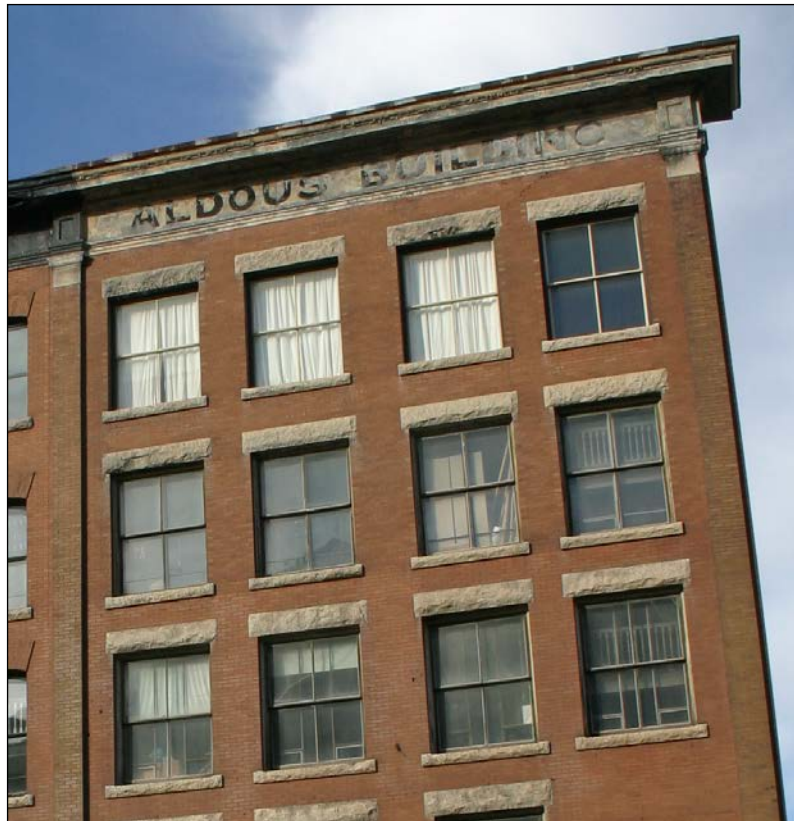
Plate 6 – Aldous Building, 376 Donald Street, front (east) façade, “ALDOUS BUILDING” signage, 2005. (M. Peterson, 2005.)
