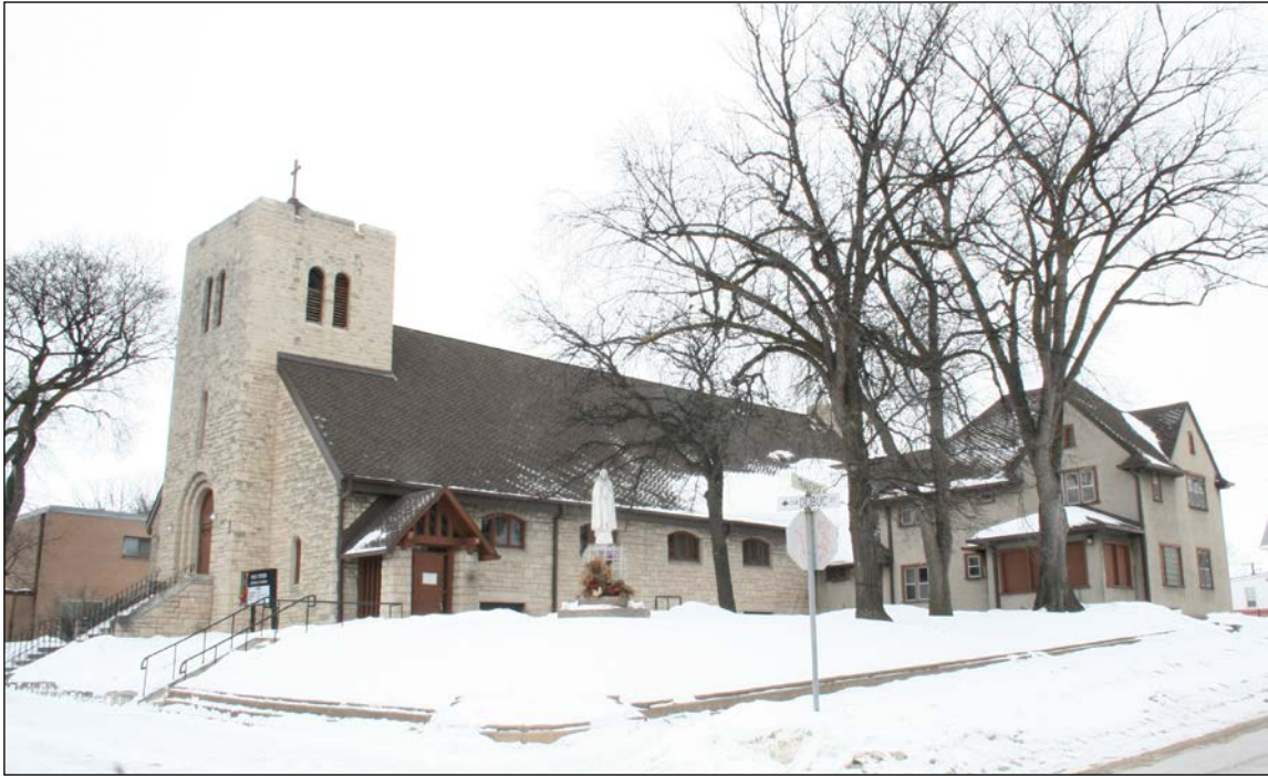
Front (north) and west façades, 2009
