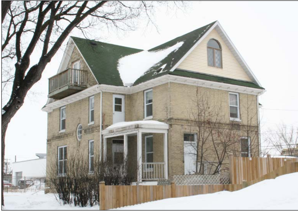
Front (north) and west façades, 2009
