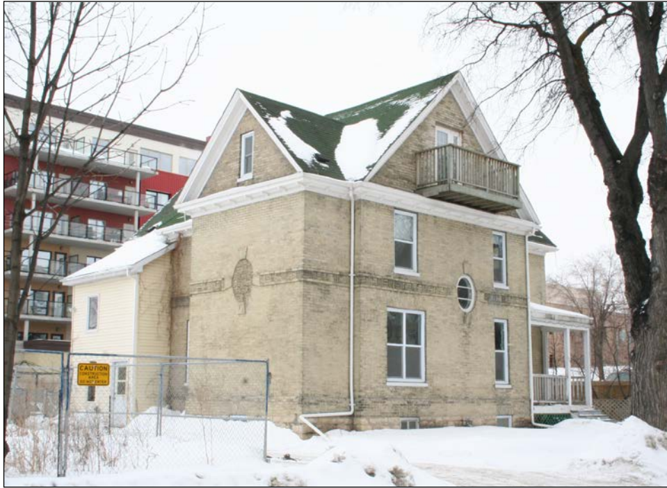
Front (north) and east façades, 2009
