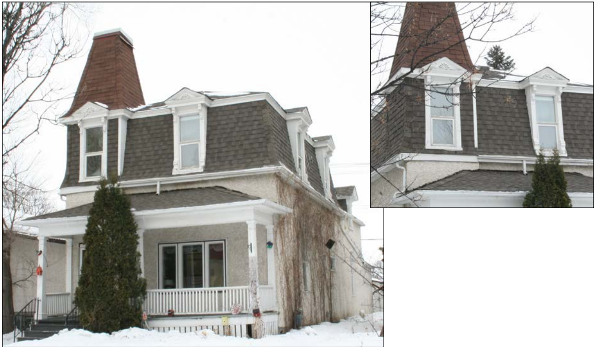
Front (south) and east façades and detail of roof, 2009
