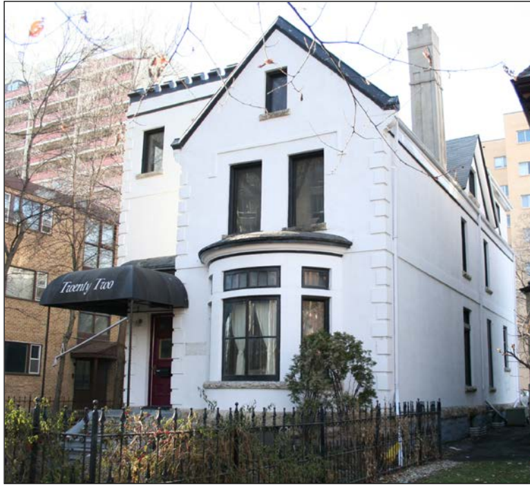
Front (east) and north façades, 2006
