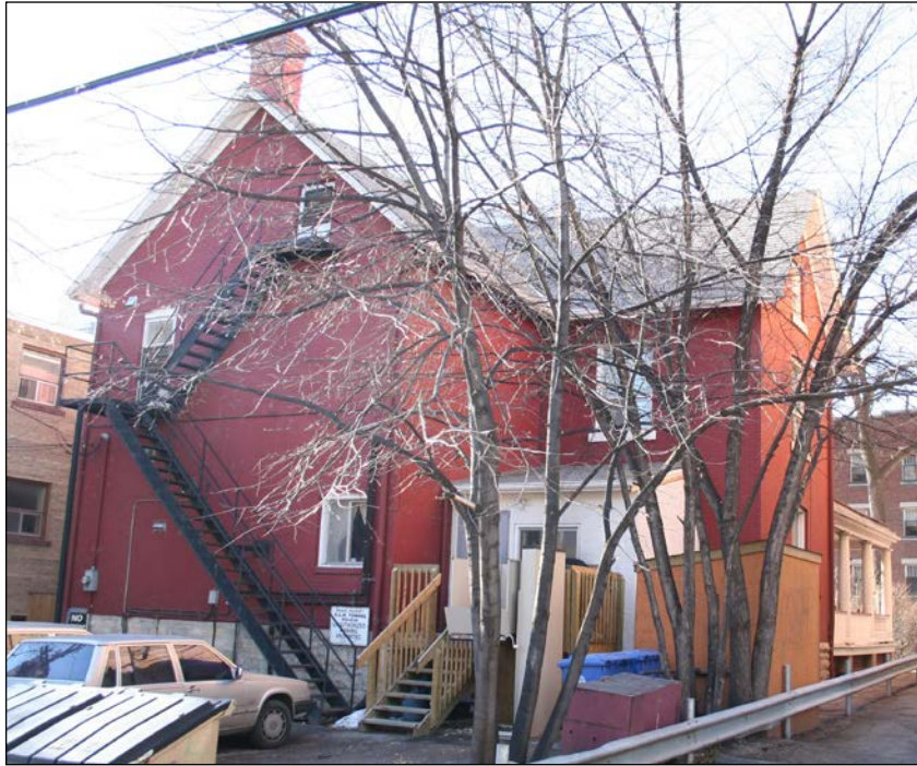
Rear (east) and north façades, 2006
