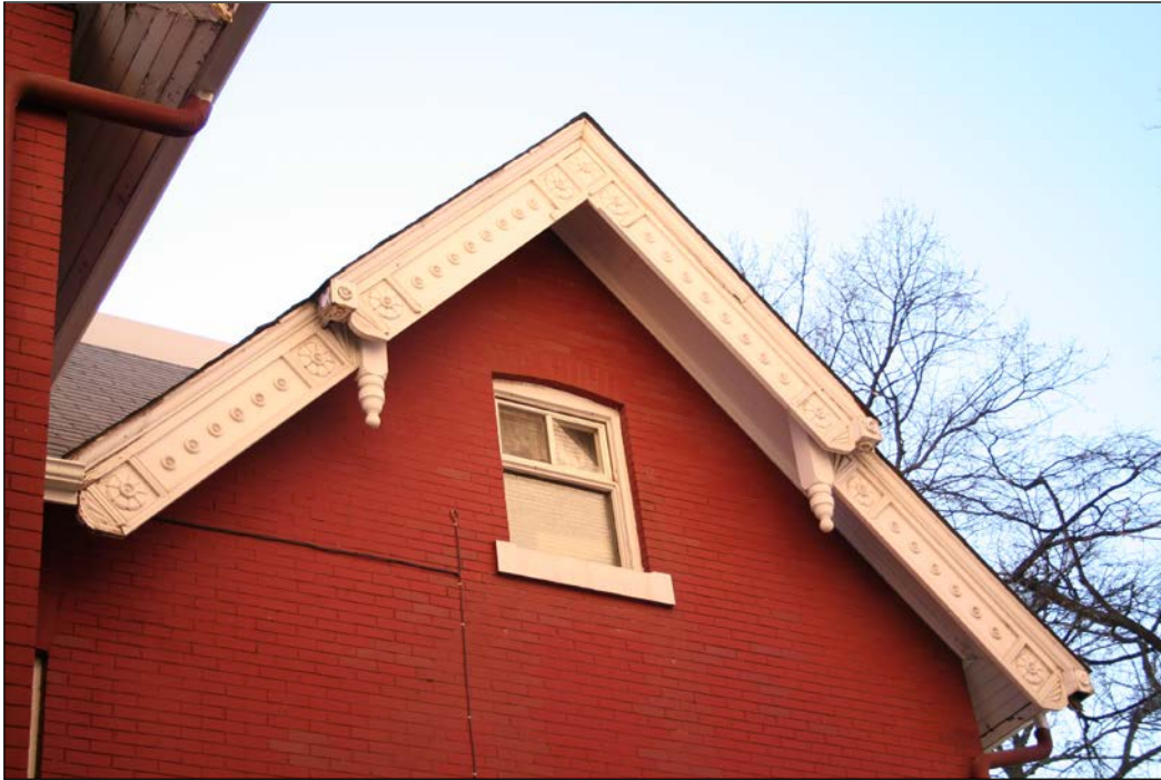
Detail of ornamental bargeboard, north side, 2006
