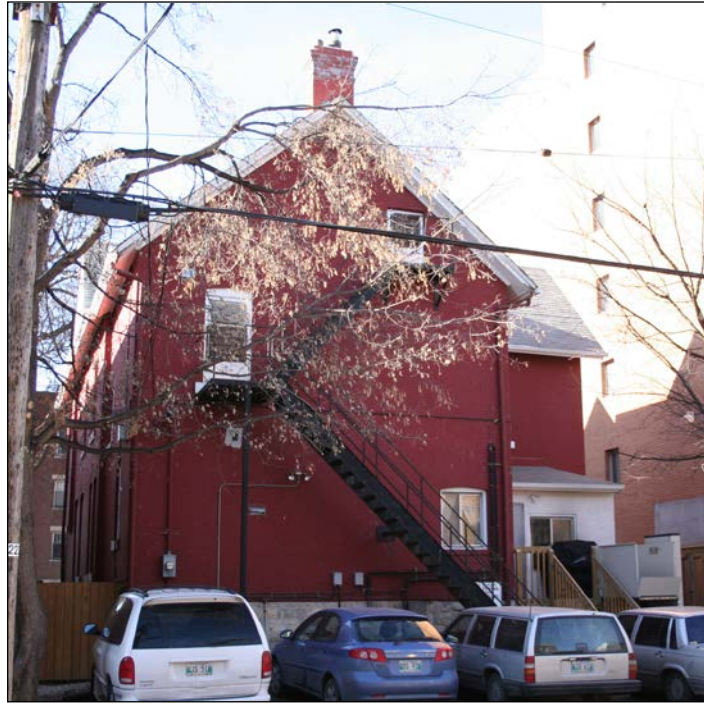
Rear (east) and south façades, 2006
