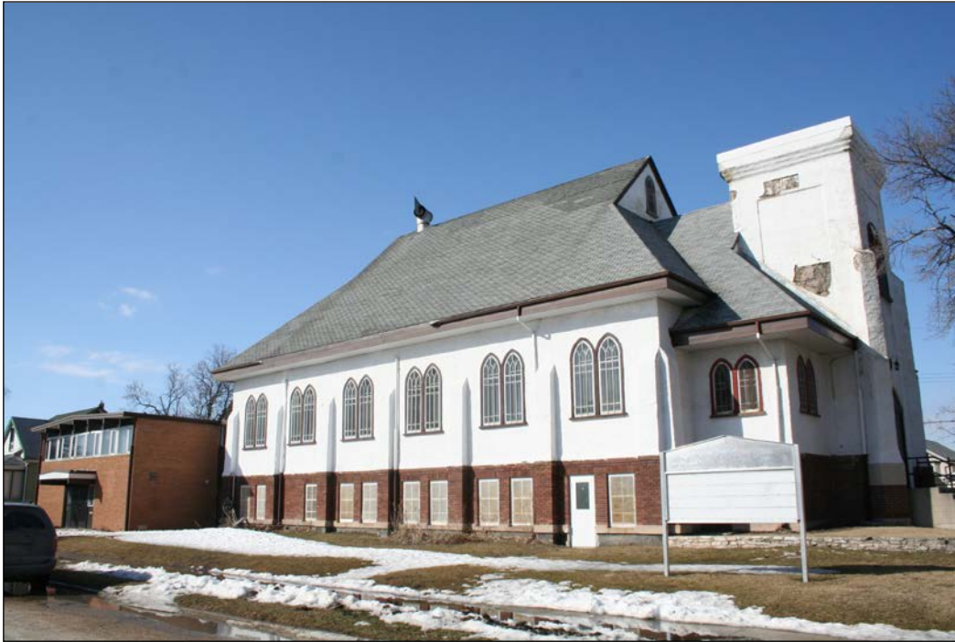
Front (east) and south façades, 2009
