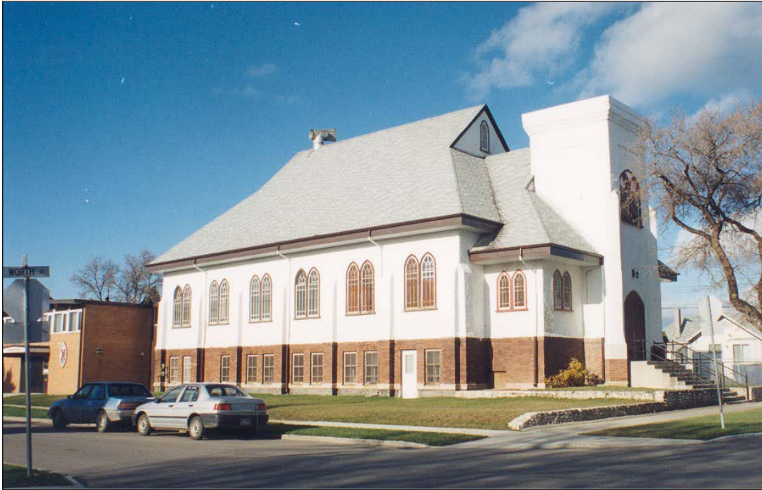
Front (east) and south façades, 1994
