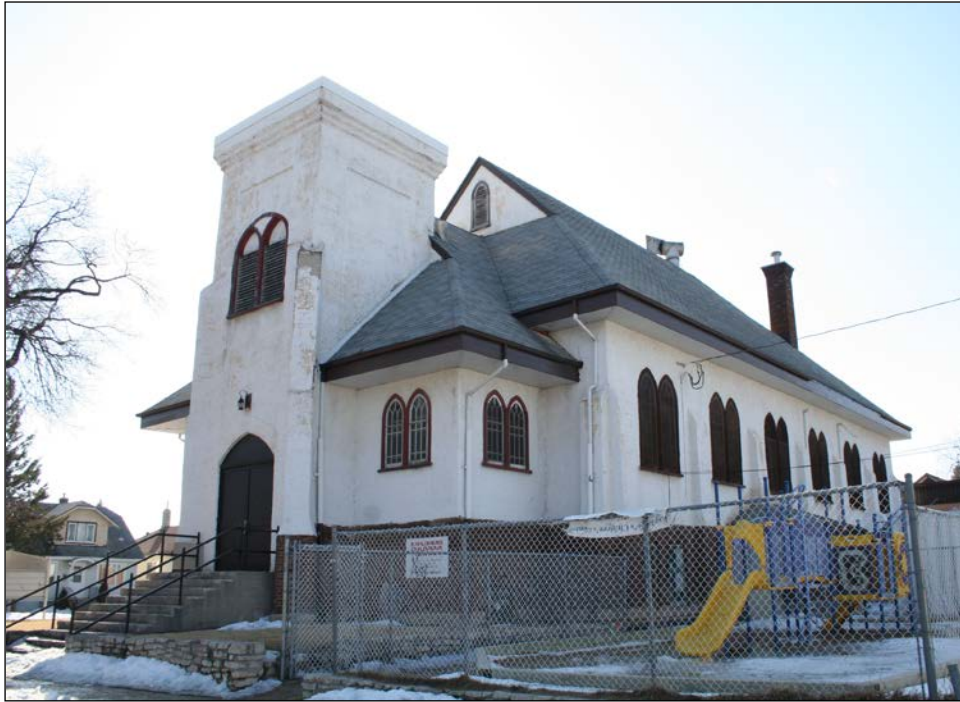
Front (east) and north façades, 2009
