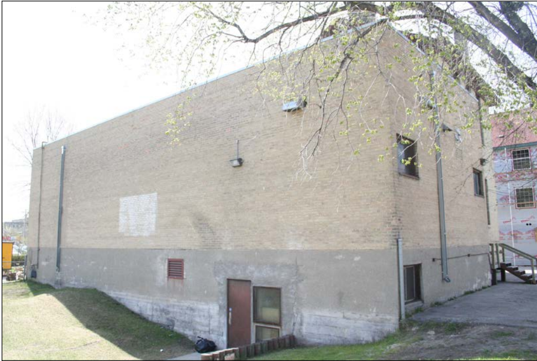
Rear (west) and north façades of addition, 2007
