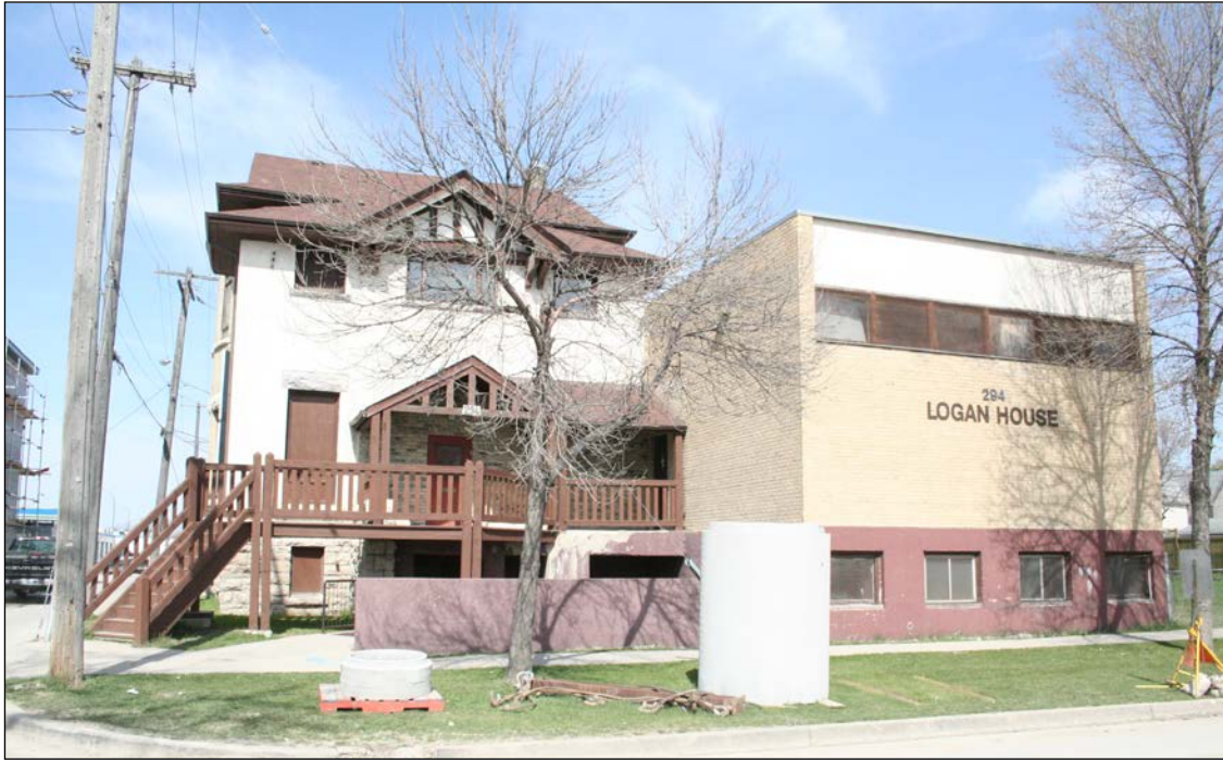
Front (east) façade and north addition, 2007
