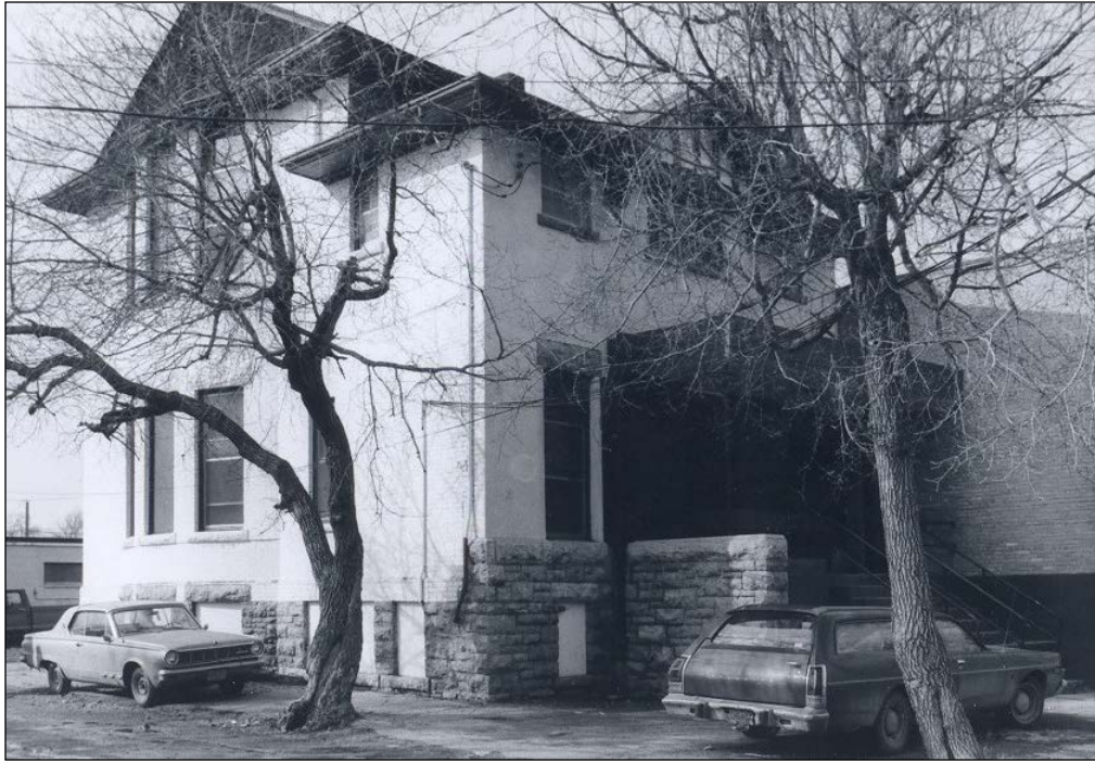
Front (east) façade, 1978
