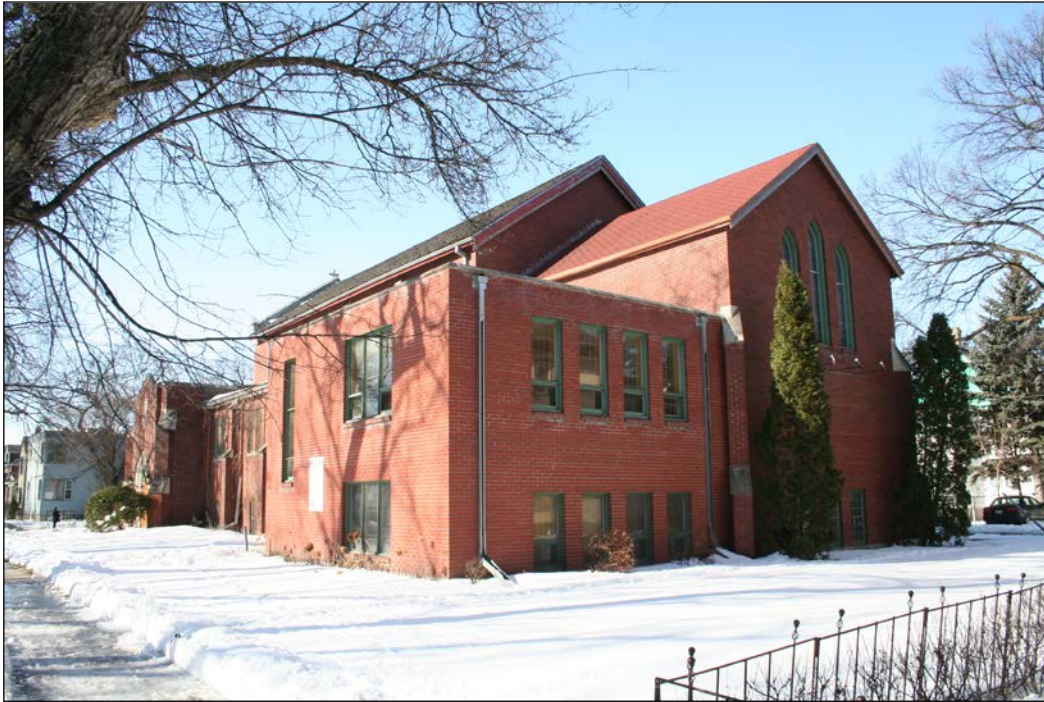
Rear (north) and east façades, 2009
