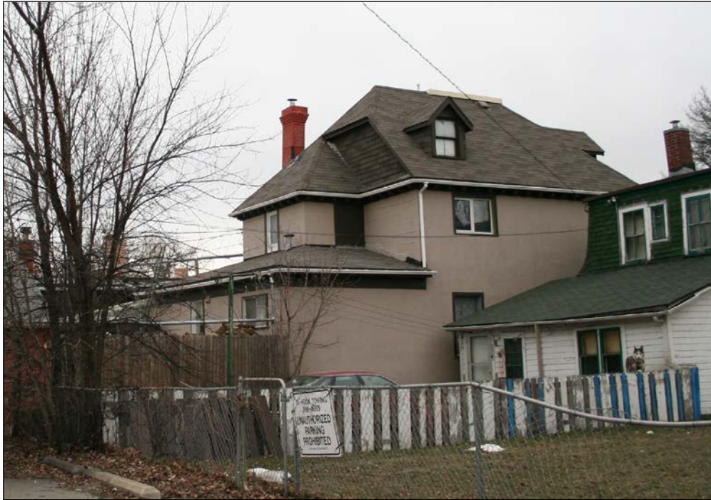
Rear (north) and west façades, 2006
