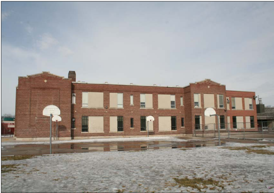
Rear (east) façade, 2009
