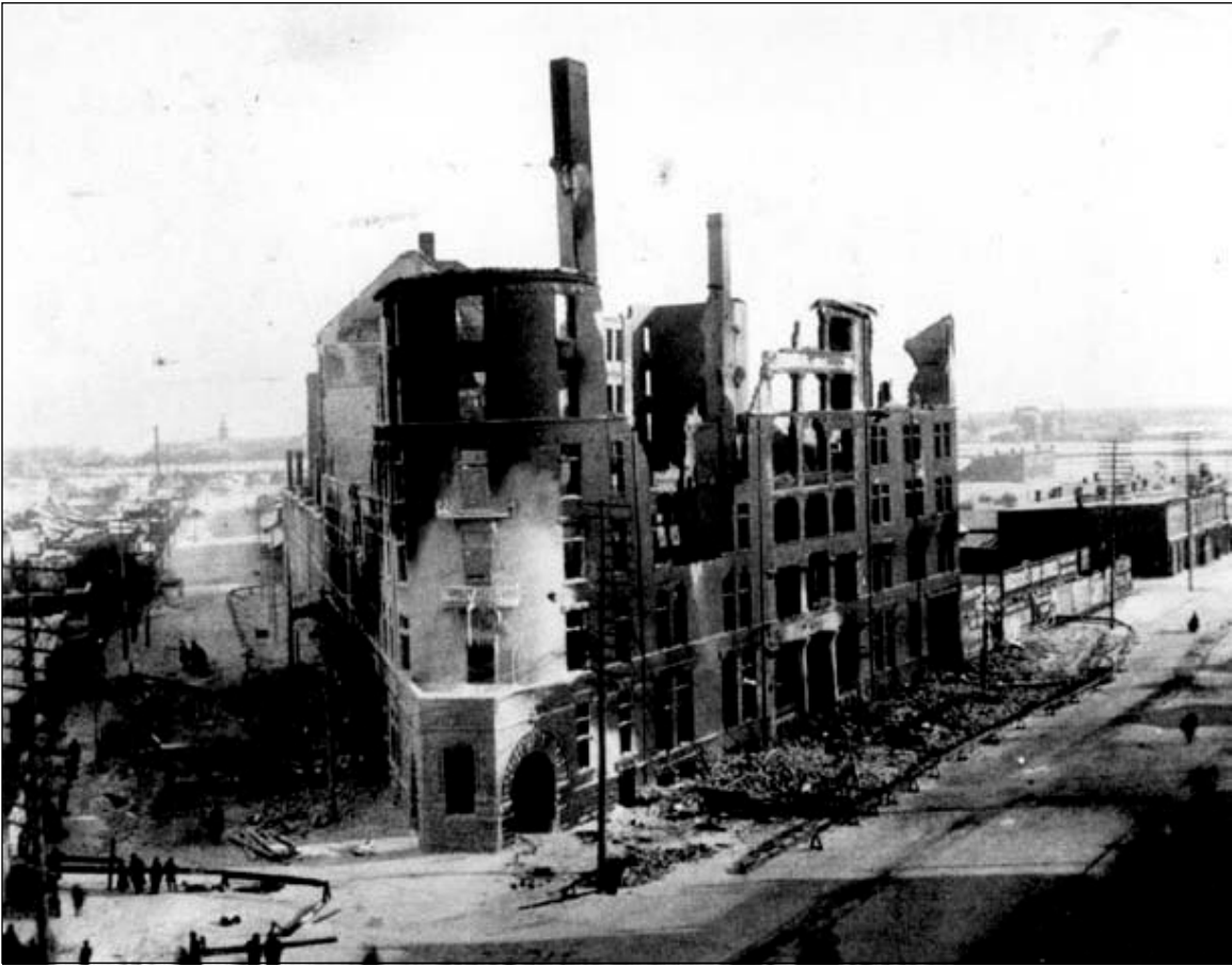
Plate 6 – Manitoba Hotel, completely destroyed by fire on February 7, 1899. ( University of Manitoba Archives, Winnipeg Tribune Collection, PC 18/7192/18-6236-123. )
