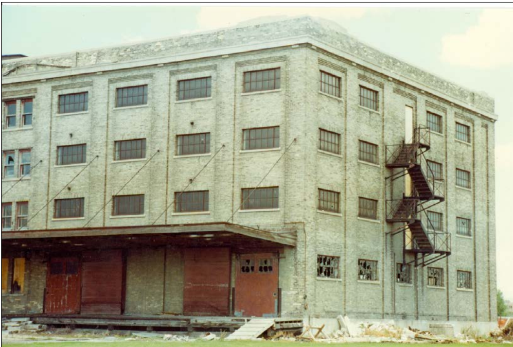
Plate 11 – Johnston Terminal Building, CNR East Yards, southwest corner, ca.1990. ( M. Peterson. )
