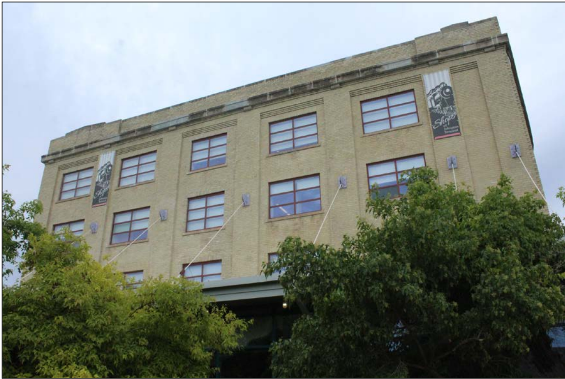
Plate 22 – Johnston Terminal Building, 25 Forks Market Road, south façade, 2019. ( M. Peterson, 2019. )
