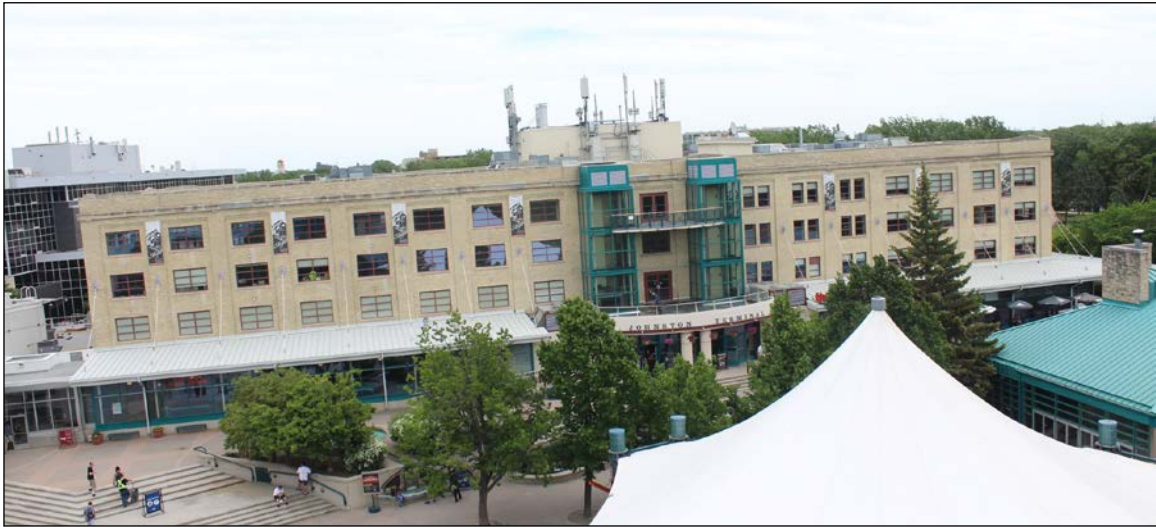
Plate 19 – Johnston Terminal Building, 25 Forks Market Road, west façade, 2019. (M. Peterson, 2019.)
