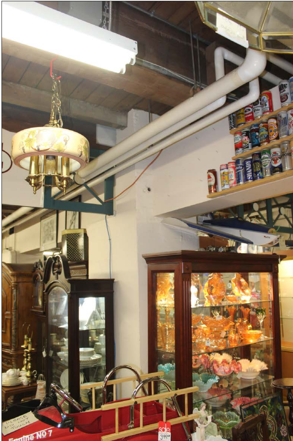
Plate 15 – Johnston Terminal Building, 25 Forks Market Road, basement retail space, showing concrete and steel support system, 2019. (M. Peterson, 2019.)
