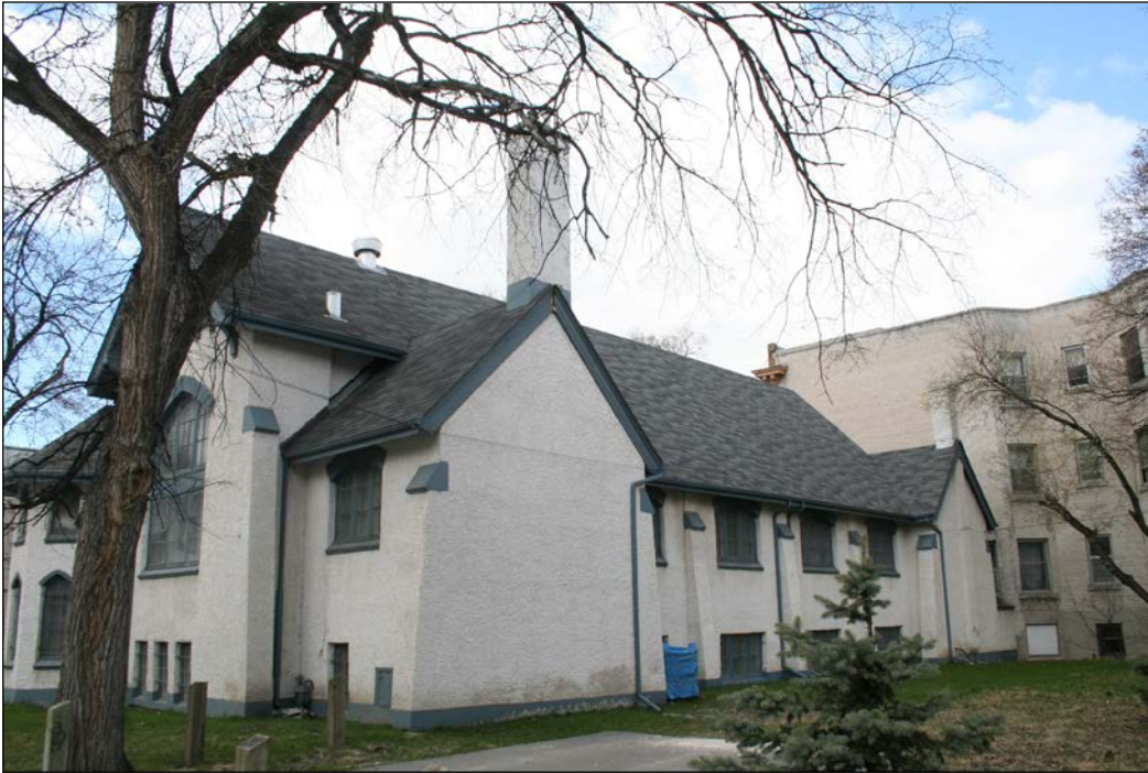
Rear (east) and south façades, 2009
