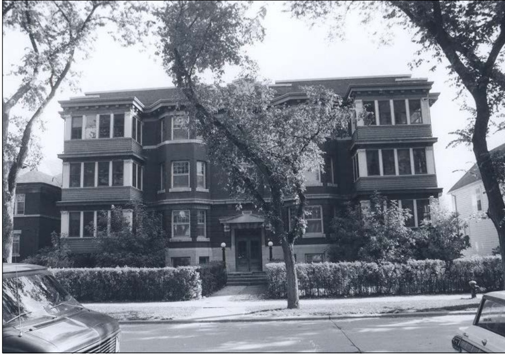
Front (west) façade, 1978
