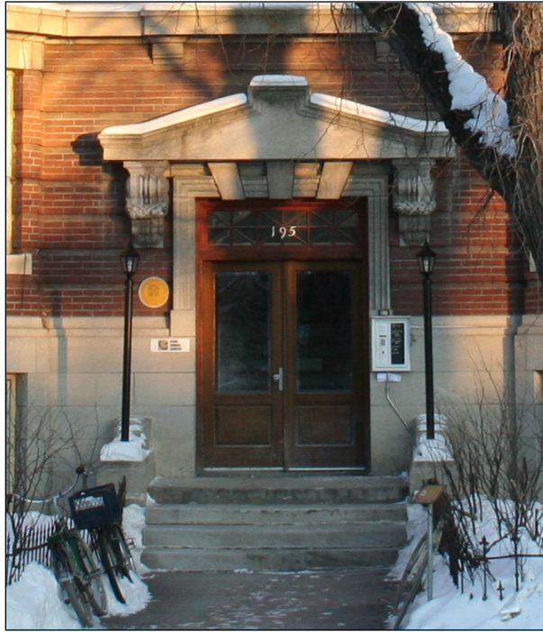
Detail of front (west) entrance, 2009
