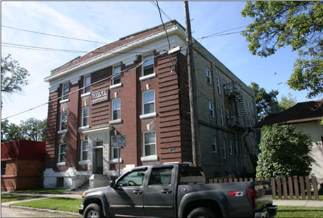
Front (east) and north façades, 2009
