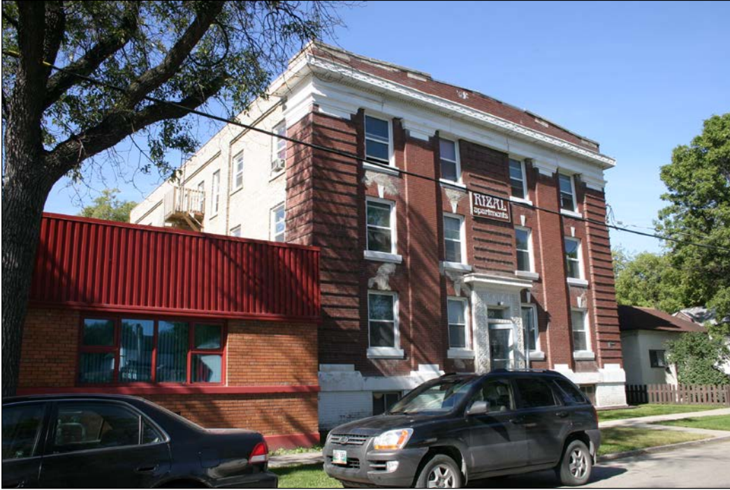
Front (east) and south façades, 2009
