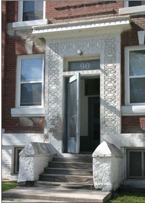
Front (east) façade detail, 1978
